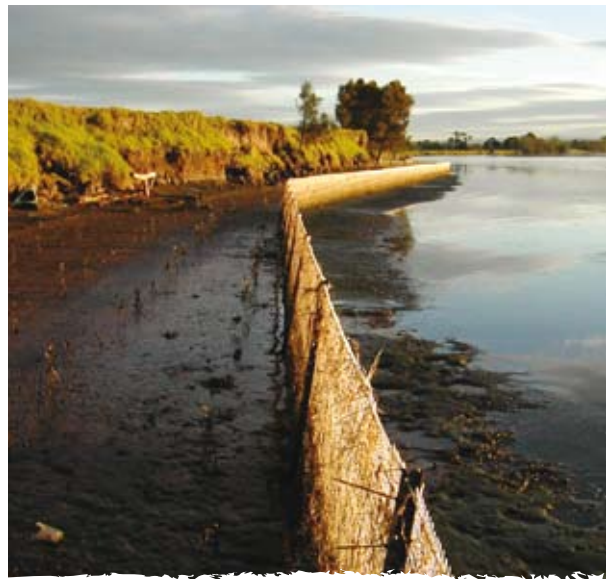
Mangrove seedlings planted in front of an eroding bank along the Shoalhaven River, with the use of temporary mesh fencing as a wave barrier. Photo: Allan Lugg, Department of Primary Industries.
