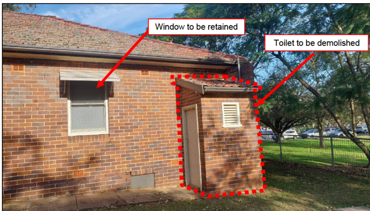
Figure 6 External toilet to be demolished (Red outline emphasis added)
