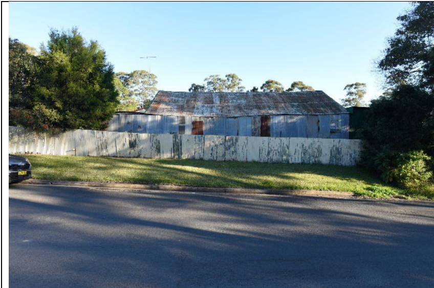
Caption: Barn at No. 24 Greenway Crescent, Windsor (exterior) Photographer: S. Johnson Copyright Owner: Lucas Stapleton Johnson & Partners Date: May 2023
