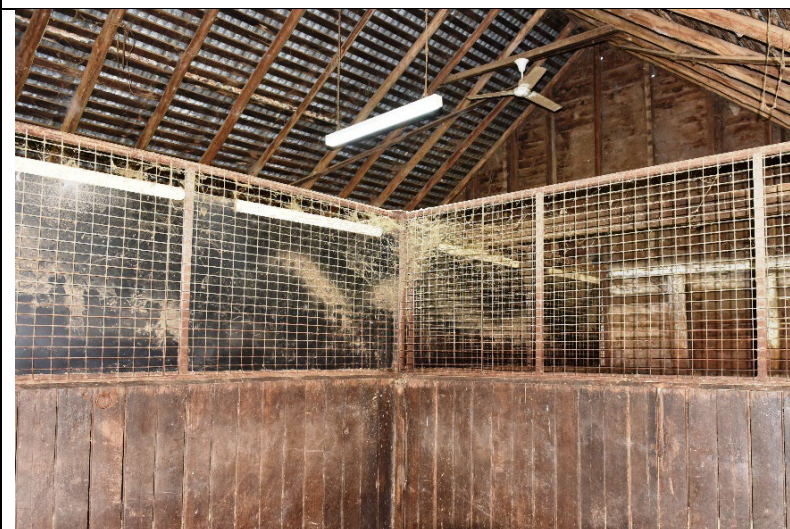
Caption: Barn 2 at 331 Hobartville, 36-40 Inalls Lane, Richmond (interior) Photographer: S. Johnson Copyright Owner: Lucas Stapleton Johnson & Partners Pty Ltd Date: June 2023
