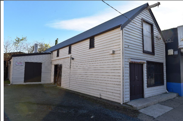
Caption: The town barn at No. 239 Windsor, Richmond (exterior). Photographer: S. Johnson Copyright Owner: Lucas Stapleton Johnson & Partners Date: May 2023
