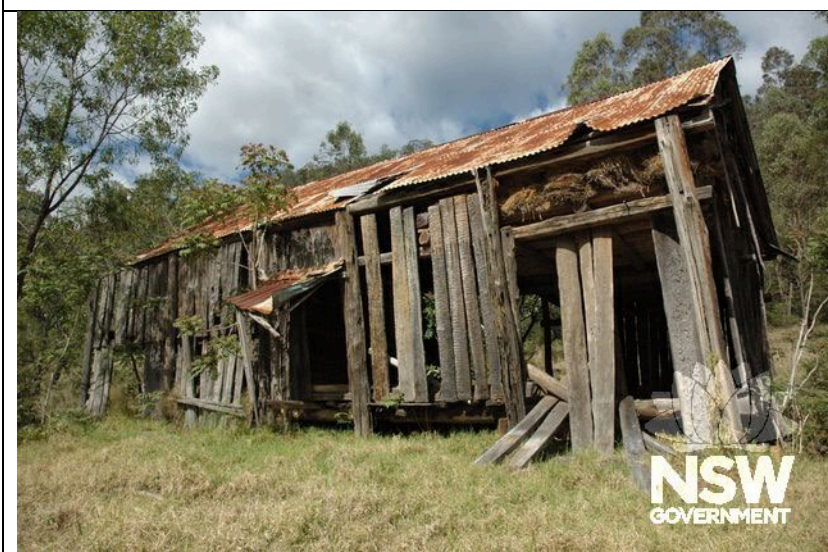
Caption: Slab barn at No. 1665 Upper Colo Road, Upper Colo. Photographer: C. Edds Copyright Owner: Graham Edds & Associates Date: 2010
