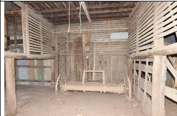
Caption: Barn at 87 Wilberforce Road, Wilberforce (interior) Photographer: S. Johnson Copyright Owner: Lucas Stapleton Johnson & Partners Pty Ltd Date: May 2023
