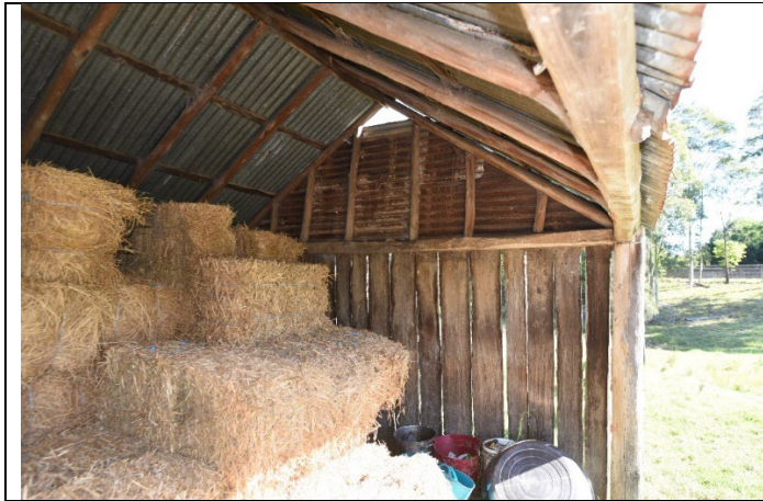
Caption: Timber slab animal shelter/hay shed at No. 10 Day Street, Windsor (interior) Photographer: S. Johnson Copyright Owner: Lucas Stapleton Johnson & Partners Pty Ltd Date: May 2023
