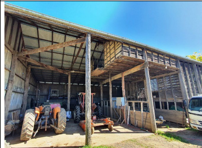
Caption: Barn at 63 Wilberforce Road, Wilberforce (interior) Photographer: S. Johnson Copyright Owner: Lucas Stapleton Johnson & Partners Date: May 2023
