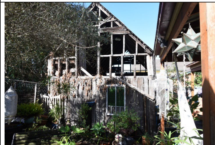
Caption: The town barn at No. 4 Catherine Street, Windsor (exterior). Photographer: S. Johnson Copyright Owner: Lucas Stapleton Johnson & Partners Date: May 2023
