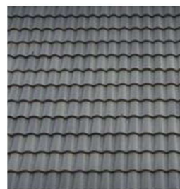
Existing Concrete Roof Tiles To Be Retained
