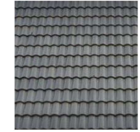
Existing Concrete Roof Tiles To Be Retained
