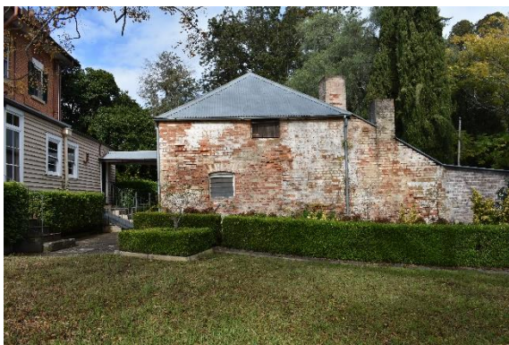
Figure 4.4 The kitchen block immediately to the west of the main house.
