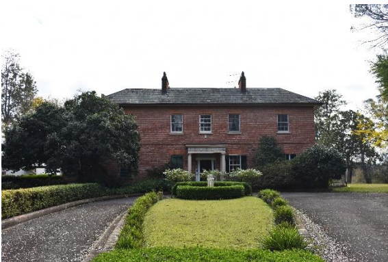
Figure 4.2 View of the entrance to the main house at Hobartville (southern elevation).
