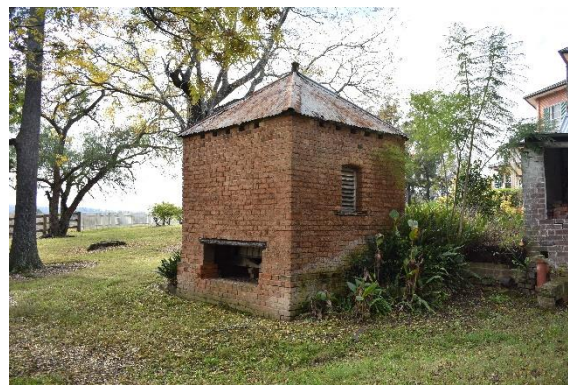
Figure 4.5 The privy adjacent to the kitchen block.
