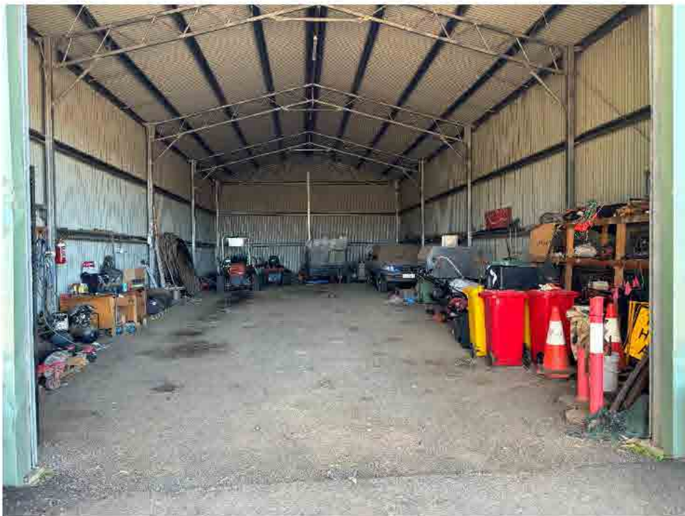
PHOTO 8 View inside the tin shed including ride-on machinery, defunct car, storage of chemicals, fuels and equipment.
