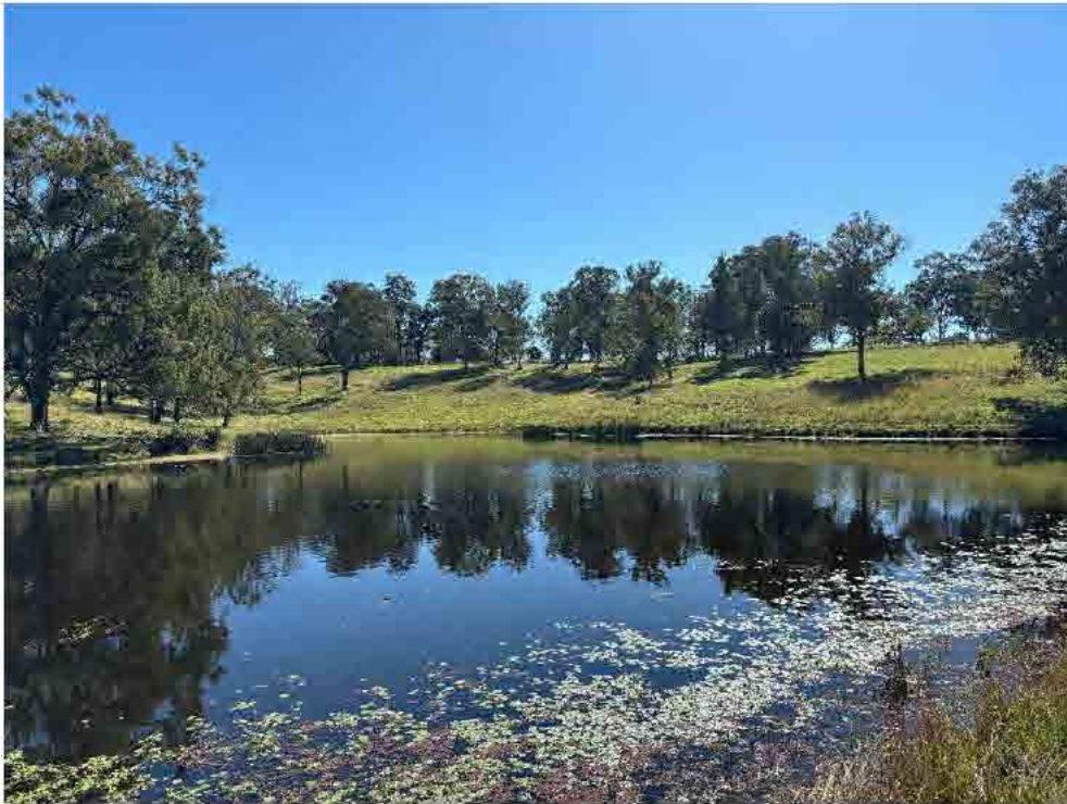
PHOTO 1 View of the dam at the southern boundary.
