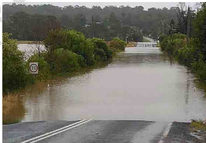
Figure 2.4 Terrace Road near Redbank Creek crossing, North Richmond, 5 July 2022 (Courtesy of a community member)
