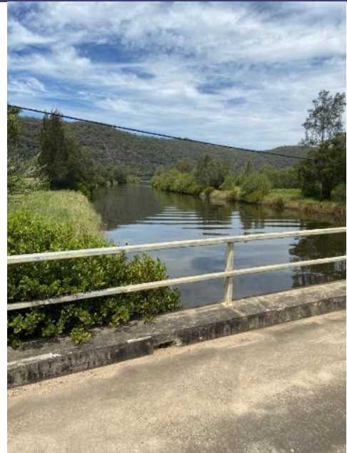
Looking upstream from bridge at Chaseling Road North, just upstream of confluence of Webbs Creek and Hawkesbury River
