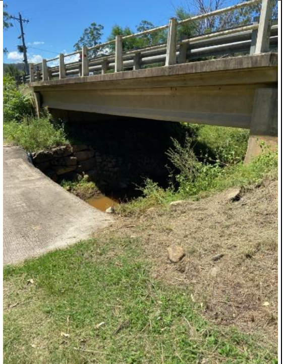
St Albans Road Bridge across Flemmings Creek
