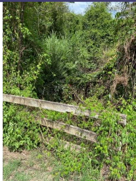
Greens Road Bridge across Greens Creek, next to Green Swamp Trail
