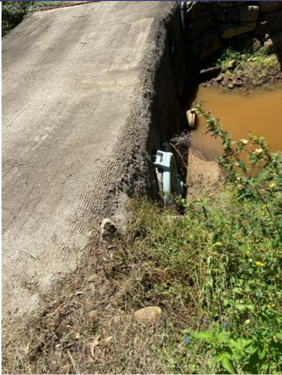
Culvert next to St Albans Road Bridge across Flemmings Creek
