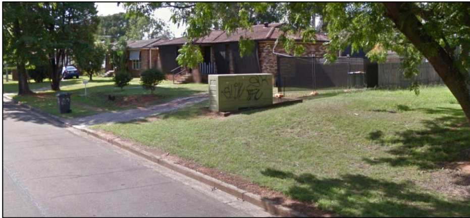
Existing Substation (S7584)
