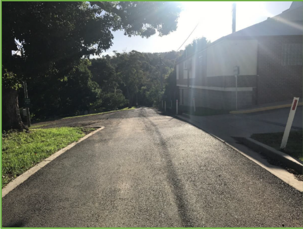
View looking west along Douglas Road showing the sealed road
