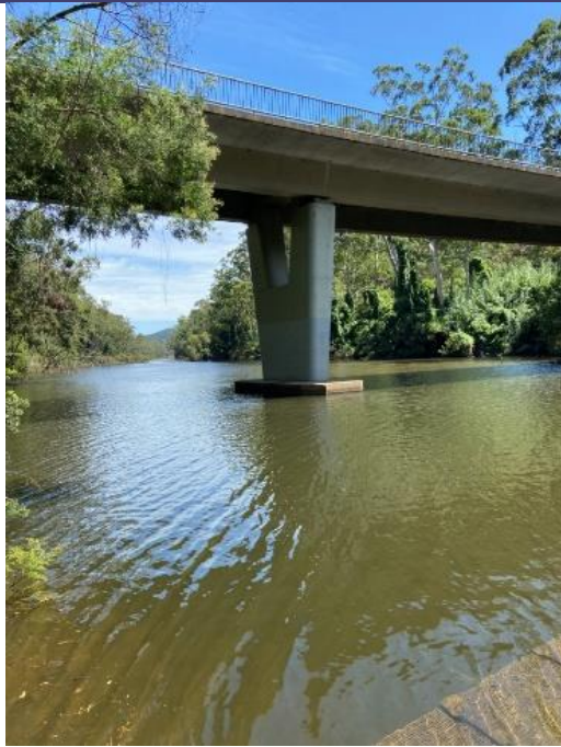
Putty Road Bridge, looking upstream
