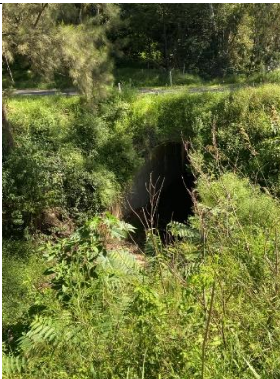
Culvert beneath Upper Colo Road connecting tributary to Upper Colo River
