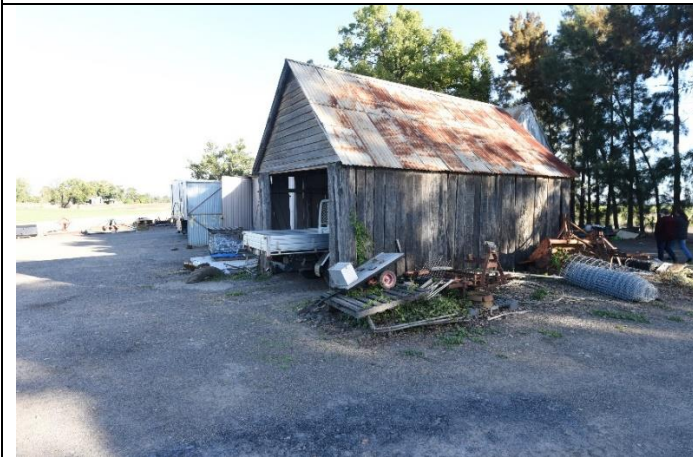
Caption: Barn B at 253 Wilberforce Road, Wilberforce (exterior) Photographer: S. Johnson Copyright Owner: Lucas Stapleton Johnson & Partners Pty Ltd Date: May 2023
