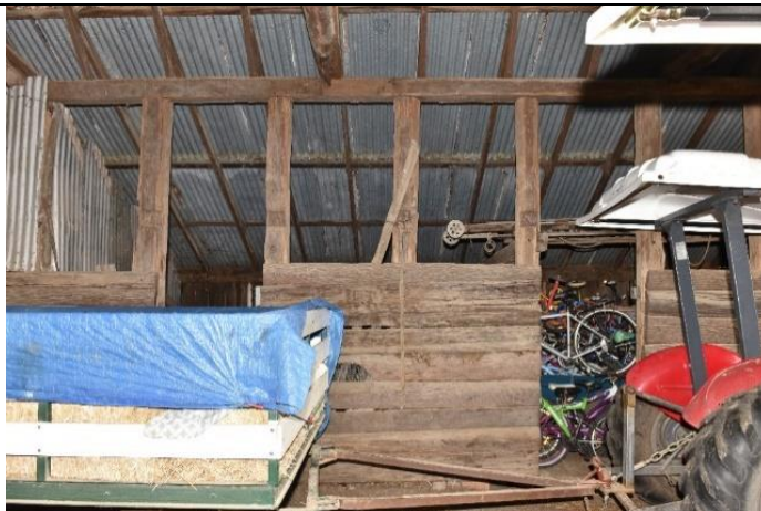
Caption: Detail of posts and beam separating main barn from skillion (note evidence of loft support), No. 496 Wilberforce Road, Wilberforce Photographer: S. Johnson Copyright Owner: Lucas Stapleton Johnson & Partners Date: July 2023
