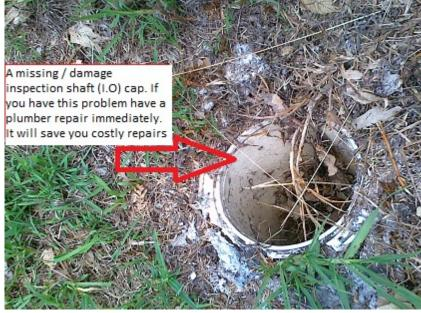
There are two ways for storm-water to get into the sewer system.
