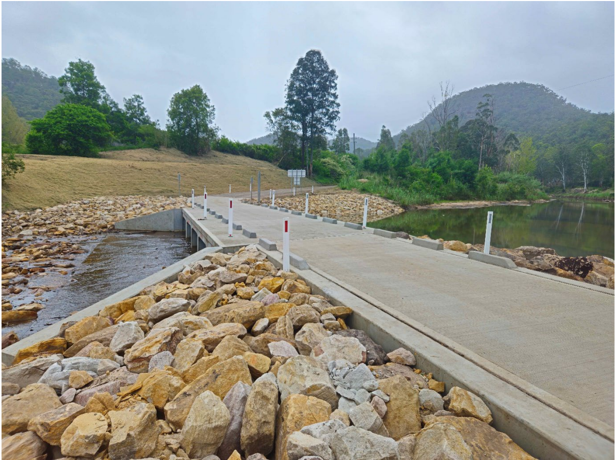
Figure 8-5 The $1.25M Gorricks Run Causeway Replacement Completed in October 2024
