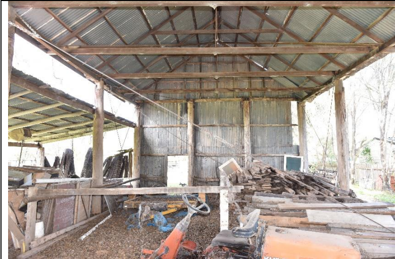
Caption: Barn 3 at 331 Hobartville, 36-40 Inalls Lane, Richmond (interior looking south) Photographer: S. Johnson Copyright Owner: Lucas Stapleton Johnson & Partners Pty Ltd Date: June 2023
