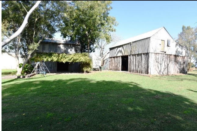
Caption: Barn A at No. 231 Pitt Town Bottoms Road, Pitt Town Bottoms (exterior) Photographer: S. Johnson Copyright Owner: Lucas Stapleton Johnson & Partners Pty Ltd Date: May 2023
