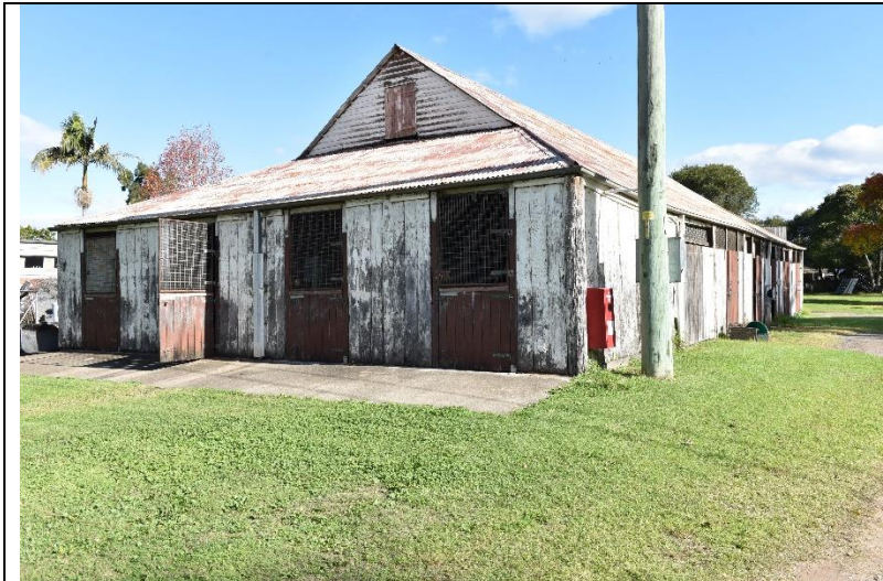
Caption: Barn 1 at 331 Hobartville, 36-40 Inalls Lane, Richmond (exterior) Photographer: S. Johnson Copyright Owner: Lucas Stapleton Johnson & Partners Pty Ltd Date: June 2023
