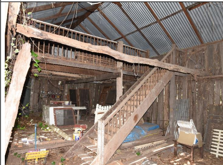
Caption: Barn 2 at No. 20-22 Buckingham Street, Pitt Town (interior) Photographer: S. Johnson Copyright Owner: Lucas Stapleton Johnson & Partners Date: May 2023
