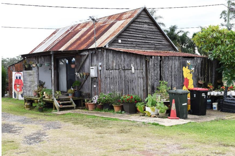
Caption: Barn at 307 Kurmond Road, Freemans Reach Photographer: S. Johnson Copyright Owner: Lucas Stapleton Johnson & Partners Pty Ltd Date: June 2023
