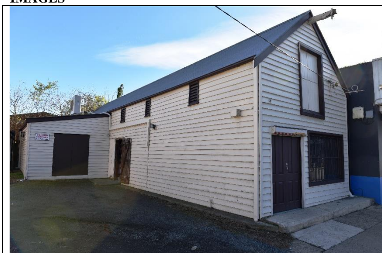
Caption: The town barn at No. 239 Windsor, Richmond (exterior). Photographer: S. Johnson Copyright Owner: Lucas Stapleton Johnson & Partners Date: May 2023
