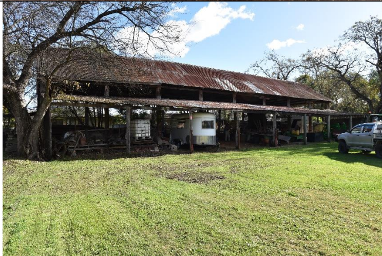
Caption: Barn 3 at 331 Hobartville, 36-40 Inalls Lane, Richmond (exterior) Photographer: S. Johnson Copyright Owner: Lucas Stapleton Johnson & Partners Pty Ltd Date: June 2023
