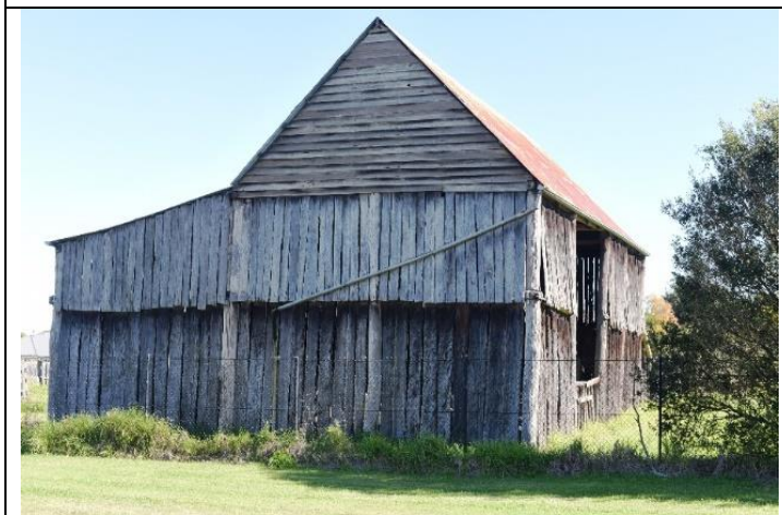
Caption: Barn A at Bona Vista complex Photographer: S. Johnson Copyright Owner: Lucas Stapleton Johnson & Partners Date: May 2023
