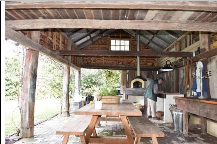
Caption: The town barn at No. 102 Lennox Street, Richmond (interior). Photographer: S. Johnson Copyright Owner: Lucas Stapleton Johnson & Partners Date: May 2023
