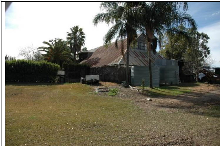
Caption: Barn B at No. 265 Pitt Town Bottoms Road, Pitt Town Bottoms Photographer: C. Edds Copyright Owner: Grahams Edds & Associates Date: 2009
