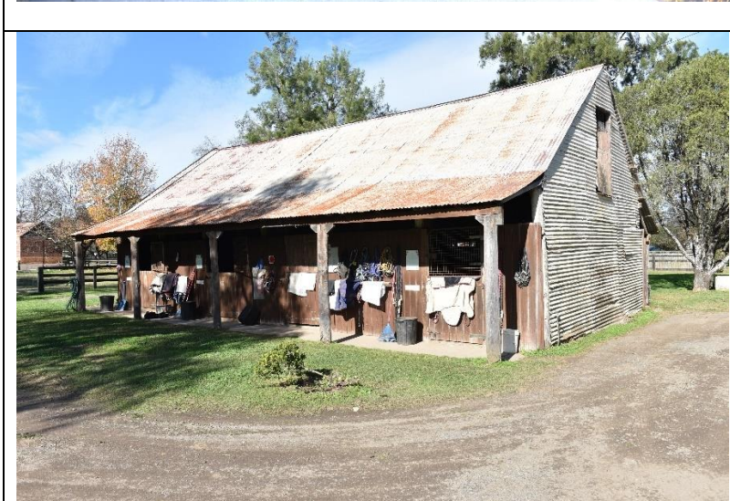
Caption: Barn 2 at 331 Hobartville, 36-40 Inalls Lane, Richmond (exterior) Photographer: S. Johnson Copyright Owner: Lucas Stapleton Johnson & Partners Pty Ltd Date: June 2023
