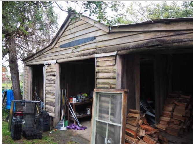
Caption: Reconstructed barn at No. 1269 Bells Line of Road, Kurrajong Heights (exterior) Photographer: S. Johnson Copyright Owner: Lucas Stapleton Johnson & Partners Date: June 2023
