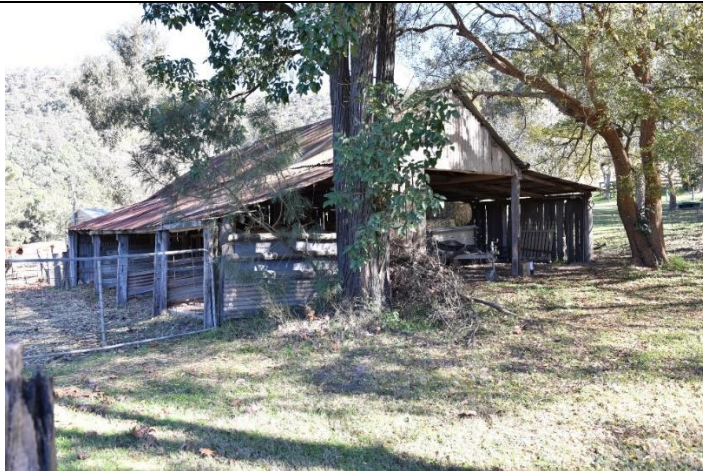
Caption: Milking Shed at No. 239 Upper Macdonald Road, St Albans (exterior) Photographer: S. Johnson Copyright Owner: Lucas Stapleton Johnson & Partners Date: June 2023
