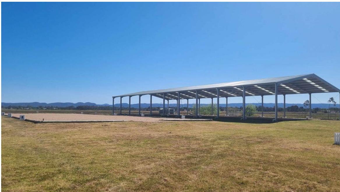
Figure 3: Existing sand arena with roof cover (right) and existing sand arena and location of proposed roof cover (left)
