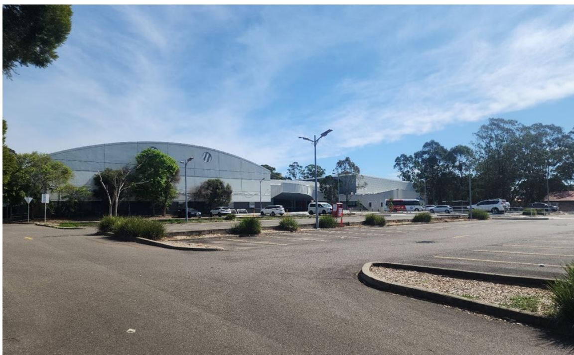
Figure 4b – View of the existing carpark towards the west (Source GAT & Associates)
