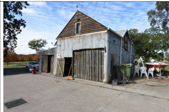
Caption: Barn at No. 251 Pitt Town Bottoms Road, Pitt Town Bottoms (exterior) Photographer: S. Johnson Copyright Owner: Lucas Stapleton Johnson & Partners Pty Ltd Date: May 2023
