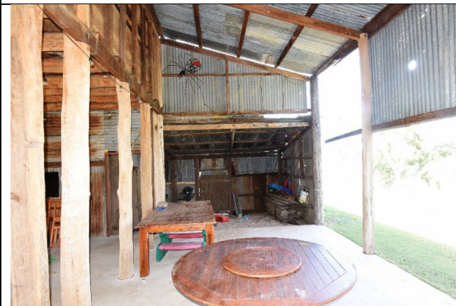
Caption: Barn A at No. 231 Pitt Town Bottoms Road, Pitt Town Bottoms (interior) Photographer: S. Johnson Copyright Owner: Lucas Stapleton Johnson & Partners Pty Ltd Date: May 2023
