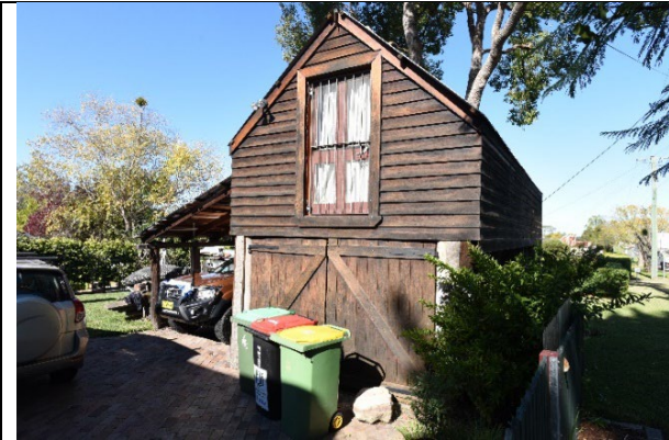
Caption: The town barn at No. 4-8 Chatham Street, Pitt Town Photographer: S. Johnson Copyright Owner: Lucas Stapleton Johnson & Partners Date: May 2023
