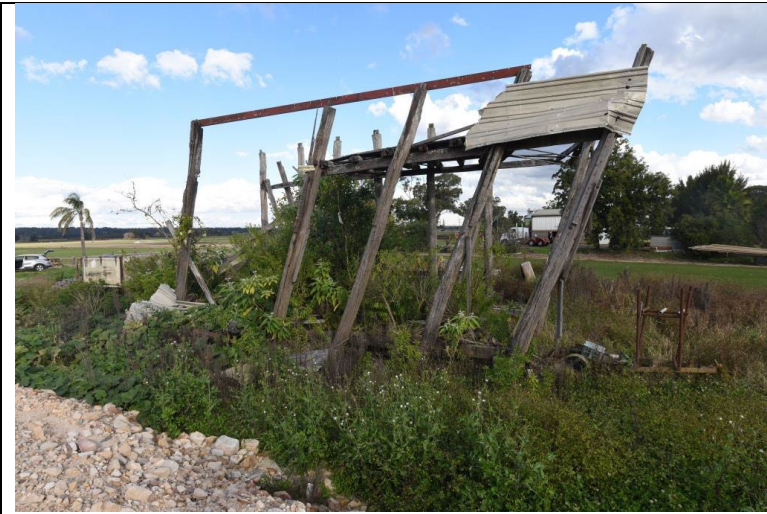
Caption: Barn at 283 Pitt Town Bottoms Road, Pitt Town Bottoms (exterior) Photographer: LSJ Copyright Owner: Lucas Stapleton Johnson & Partners Pty Ltd Date: May 2023:
