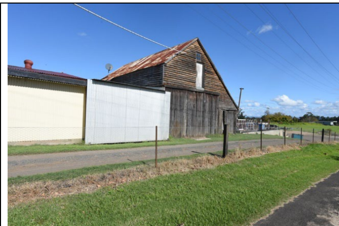
Caption: Barn at No. 313 Pitt Town Bottoms Road, Pitt Town Bottoms Photographer: S. Johnson Copyright Owner: Lucas Stapleton Johnson & Partners Date: May 2023
