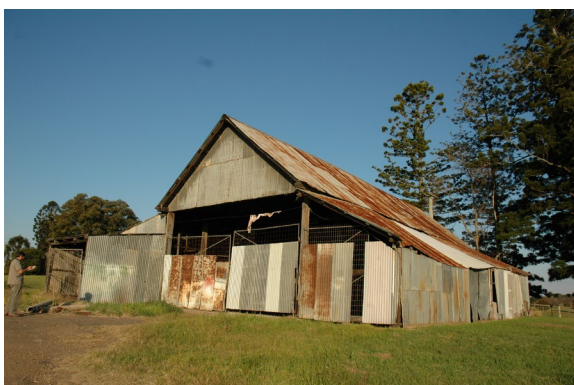
Figure 6. 5: Northern elevation of Tebbutts Barn in 2011. Source: G & C Edds
