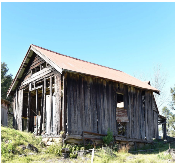
Figure 3. 33: Barn 7 at No. 135 A & B Wollombi Road, St. Albans with stone base course.
