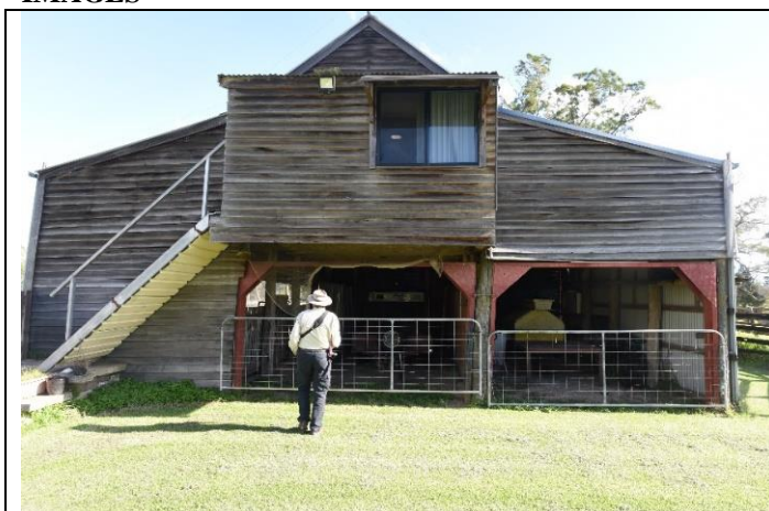
Caption: Barn at 331 Cattai Road, Cattai (exterior) Photographer: S. Johnson Copyright Owner: Lucas Stapleton Johnson & Partners Pty Ltd Date: May 2023
