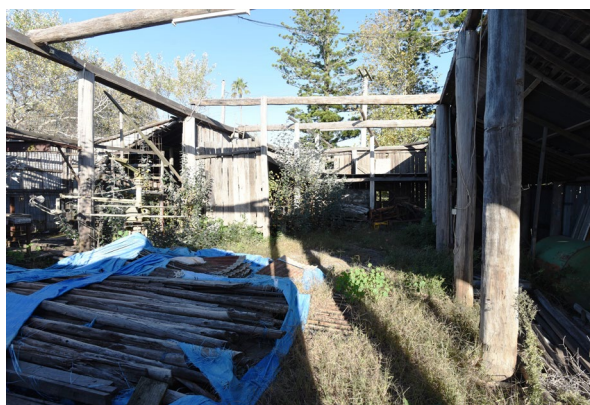
Figure 6. 10: View of interior of Tebbutt’s Barn in May 2023 showing salvaged and stored building components waiting reconstruction works.
