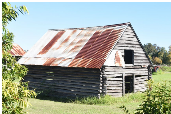
Figure 3. 21: The horizontal log outbuilding at No. 11 Amelia Grove, Pitt Town, which is possibly a corn drying shed.
