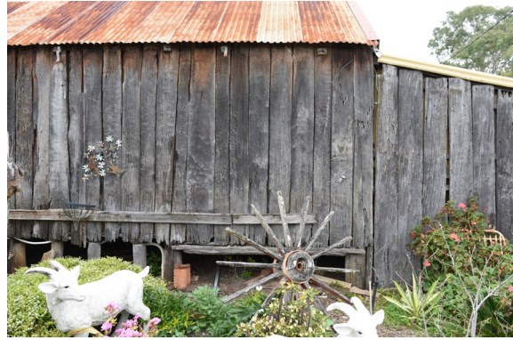
Figure 3. 36: Floor structure of barn at No. 307 Kurmond Road, Freemans Reach.
