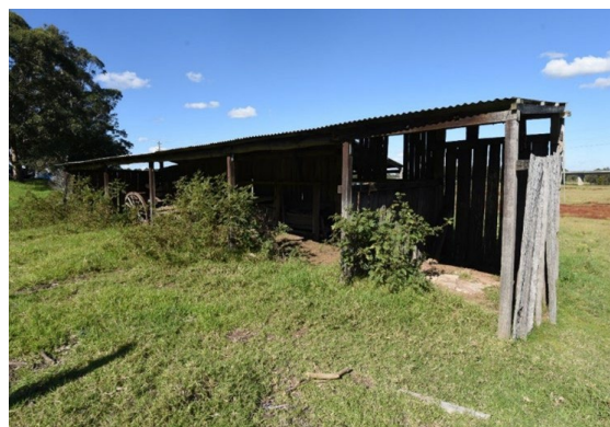
Figure 3. 20: Former milking bails and stables at No. 10 Day Street, Windsor.
