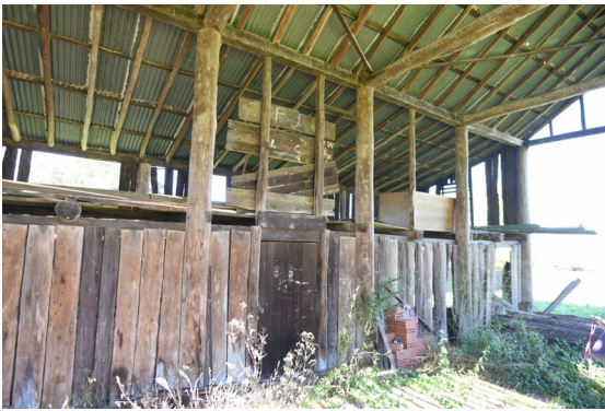
Figure 3. 37: Corn drying loft in barn at No. 26A Buckingham Street, Pitt Town
