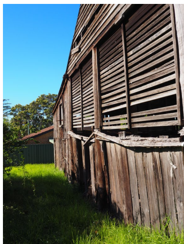
Figure 3. 29: Detail of timber vertical slabs and horizontal slats to barn at No. 26A Buckingham Street, Pitt Town.
