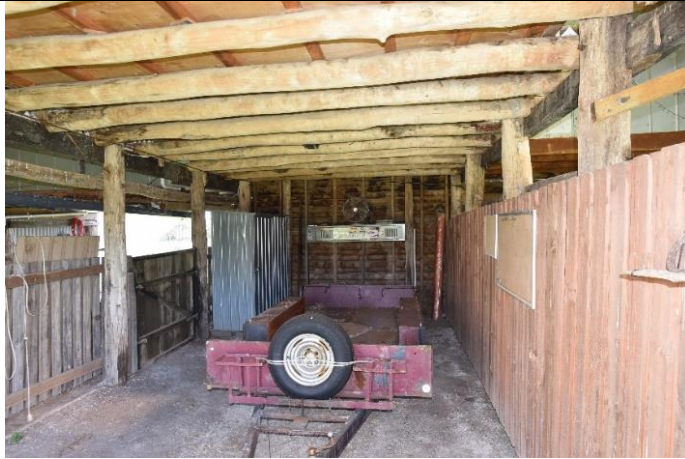
Caption: Barn at 331 Cattai Road, Cattai (interior) Photographer: S. Johnson Copyright Owner: Lucas Stapleton Johnson & Partners Pty Ltd Date: May 2023
