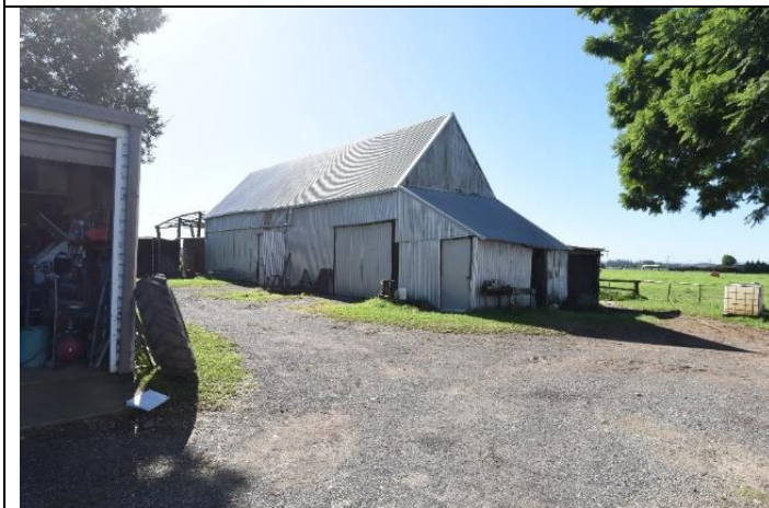
Caption: Barn B at 331 Freemans Reach Road, Freemans Reach (exterior) Photographer: LSJ Copyright Owner: Lucas Stapleton Johnson & Partners Pty Ltd Date: May 2023
