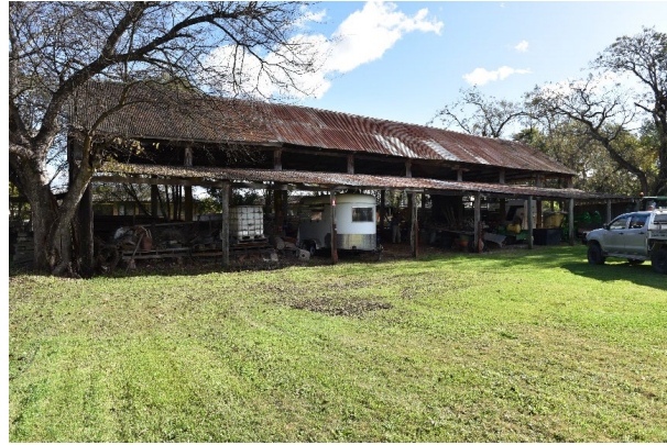
Figure 3. 13: Large barn 3 at Hobartville, No. 36-40 Inalls Lane, Richmond.
