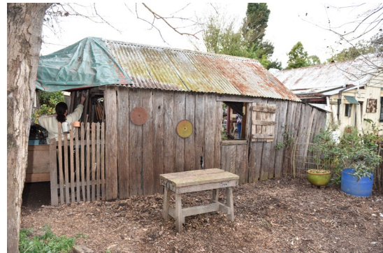
Figure 3. 11: Town barn at rear of No. 87 King Road, Wilberforce.
