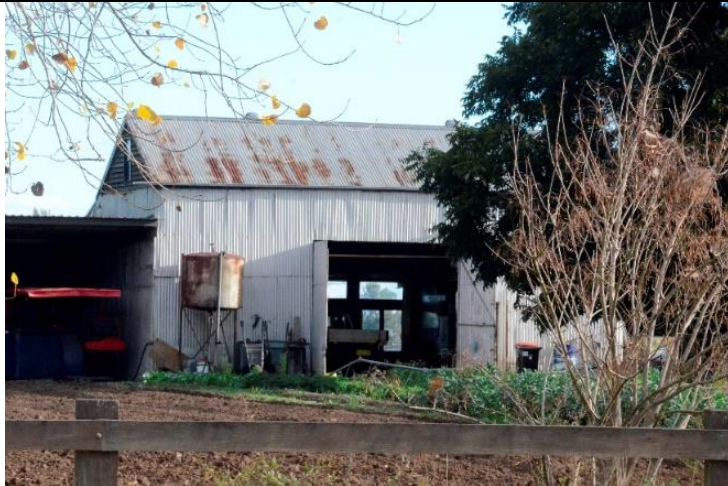
Caption: Barn at 279 Freemans Reach Road, Freemans Reach (exterior) Photographer: G. Edds Copyright Owner: Graham Edds & Associates Date: June 2023
