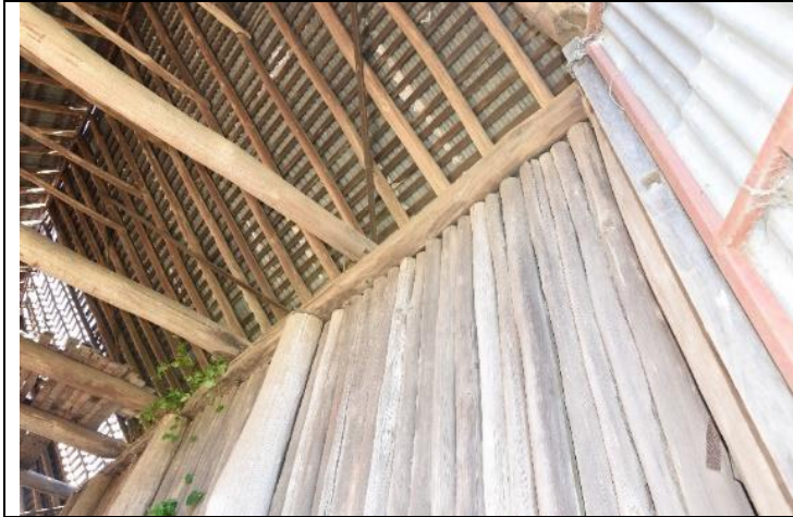
Caption: Barn at 56 Freemans Reach Road, Freemans Reach (interior)
