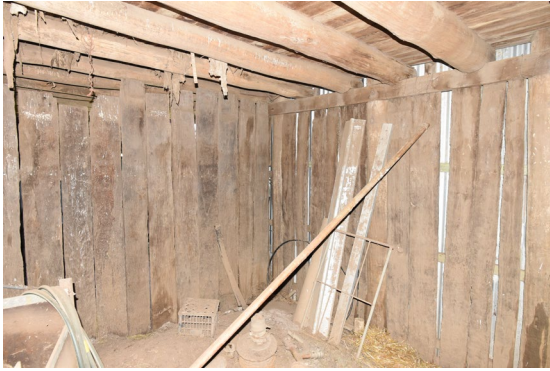
Figure 3. 31: Internal view of barn at No. 331 Freemans Reach Road, Freemans Reach with slab wall cladding and corrugated iron over externally.
