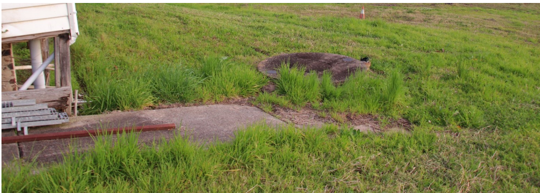
Existing septic tank/path to be removed
