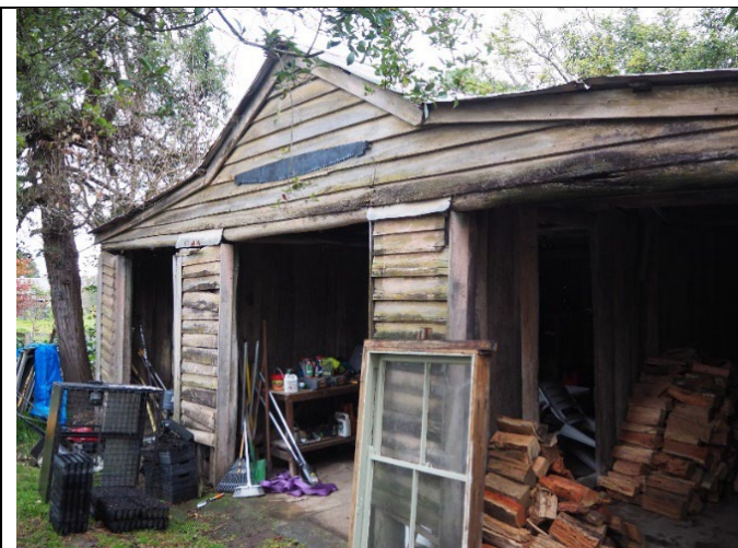
Caption: Reconstructed barn at No. 1269 Bells Line of Road, Kurrajong Heights (exterior) Photographer: S. Johnson Copyright Owner: Lucas Stapleton Johnson & Partners Date: June 2023
