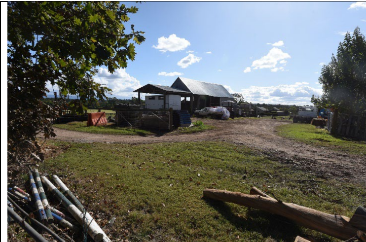
Caption: Barn at No.142 Bathurst Street, Pitt Town (exterior) Photographer: S. Johnson Copyright Owner: Lucas Stapleton Johnson & Partners Date: May 2023
