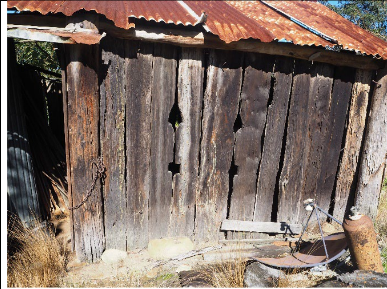
Caption: Slots for rails in slab wall of stables at 480 Laws Farm Road, Lower Portland Photographer: S. Johnson Copyright Owner: Lucas Stapleton Johnson & Partners Date: June 2023
