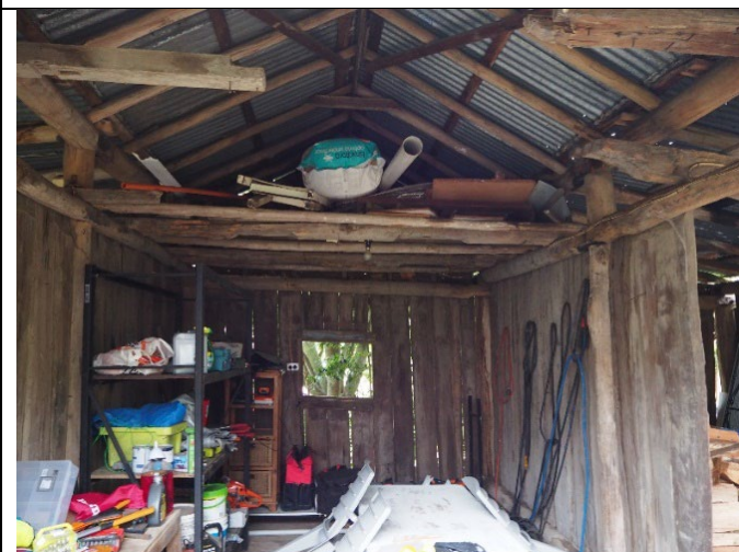
Caption: Reconstructed barn at No. 1269 Bells Line of Road, Kurrajong Heights (interior) Photographer: S. Johnson Copyright Owner: Lucas Stapleton Johnson & Partners Date: June 2023
