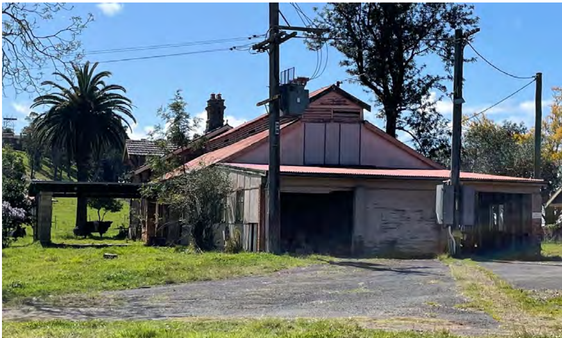
Plate 3-26: South-western elevation of Building 2 (AECOM, 2022). Compare with Plate 3-1
