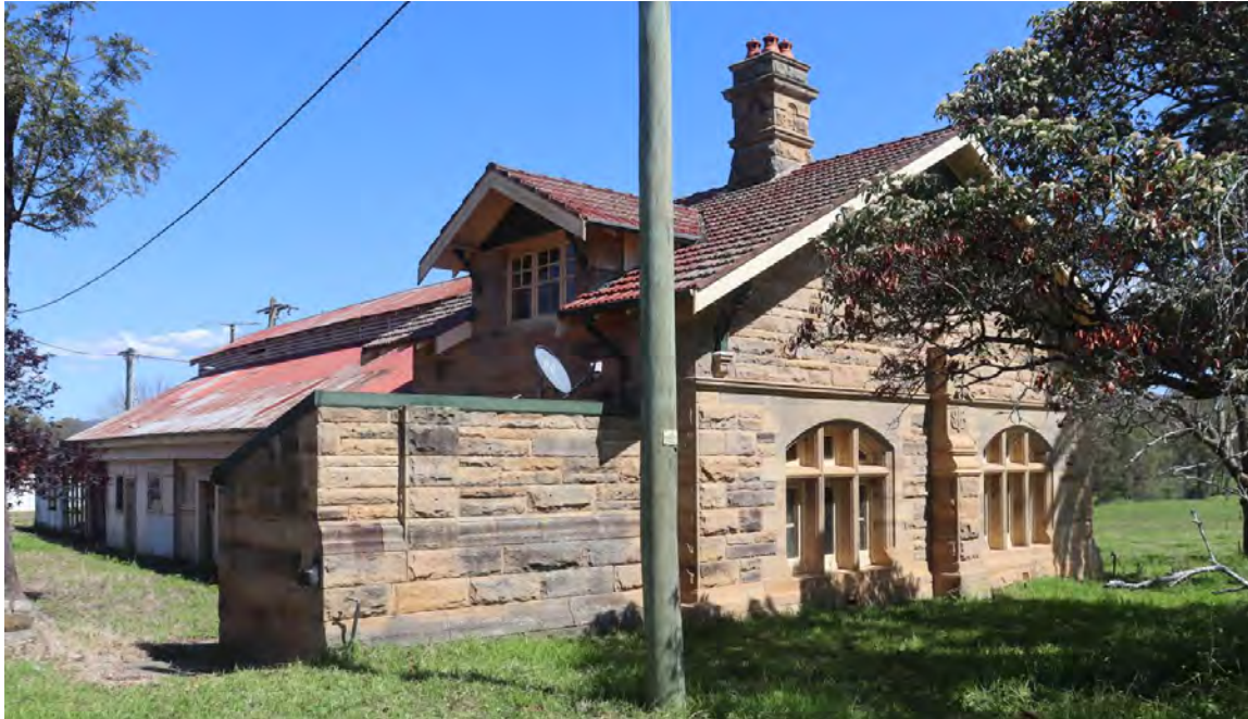
Plate 3-20: Building 2, looking south (AECOM, 2022)
