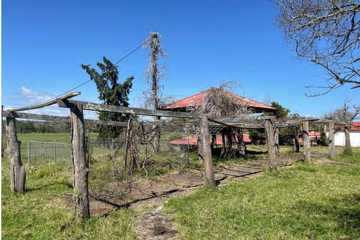
Plate 3-18: Pergola with wisteria at south of Building 1 (AECOM, 2022)
