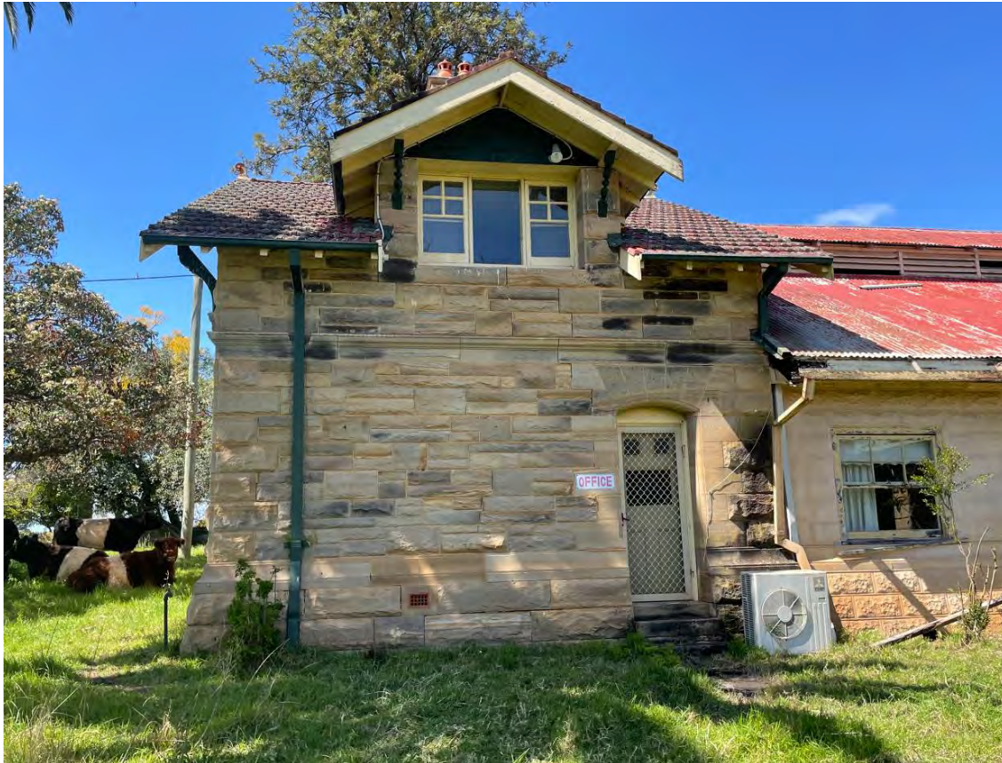
Plate 3-25: Dormer window in stone section of Building 2 (AECOM, 2022)
