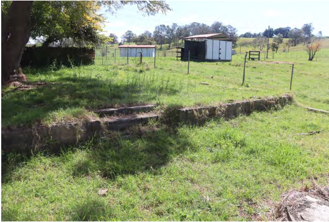
Plate 3-14: Stone retaining wall and steps. Note masonry from fountain in lower right of frame (AECOM, 2022)
