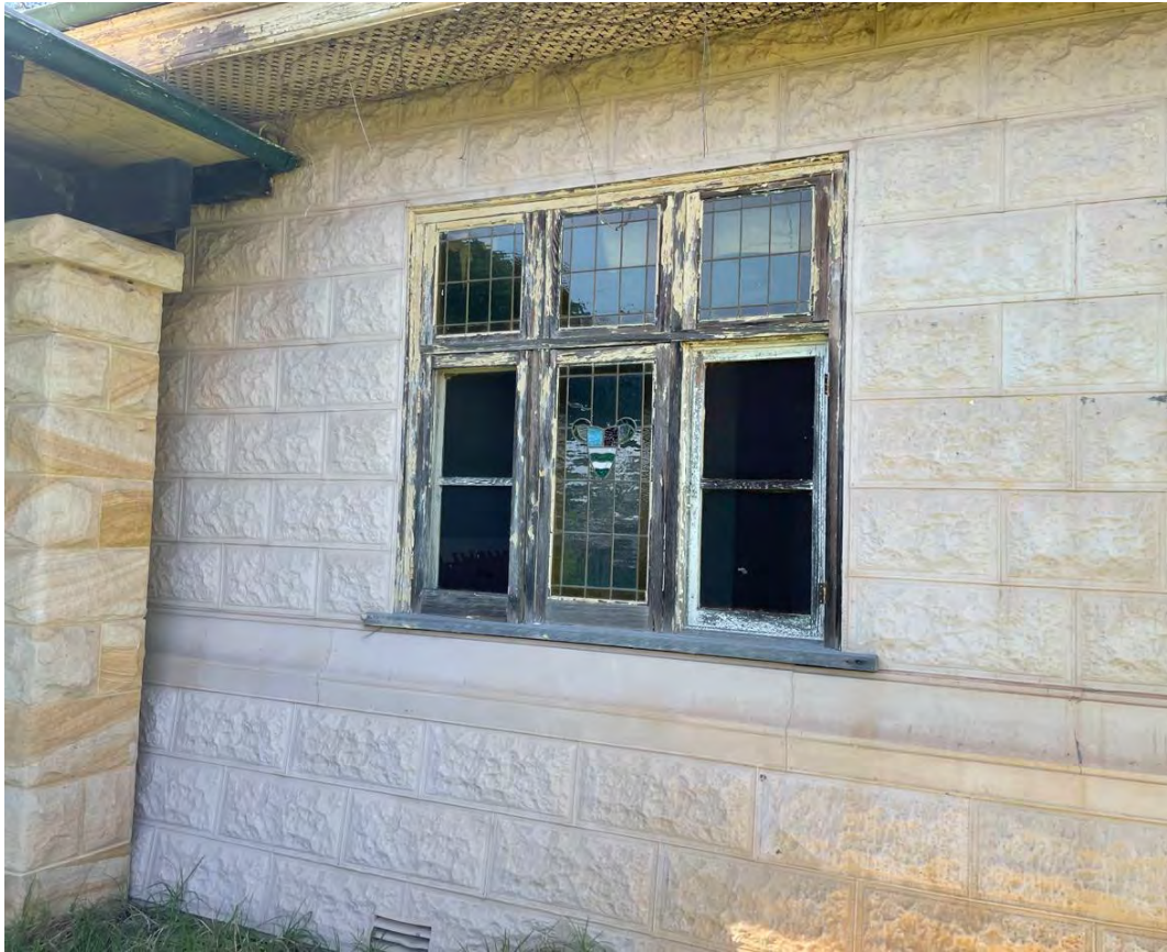
Plate 3-23: Detail of leadlight window in north western elevation of Building 2 (AECOM, 2022)
