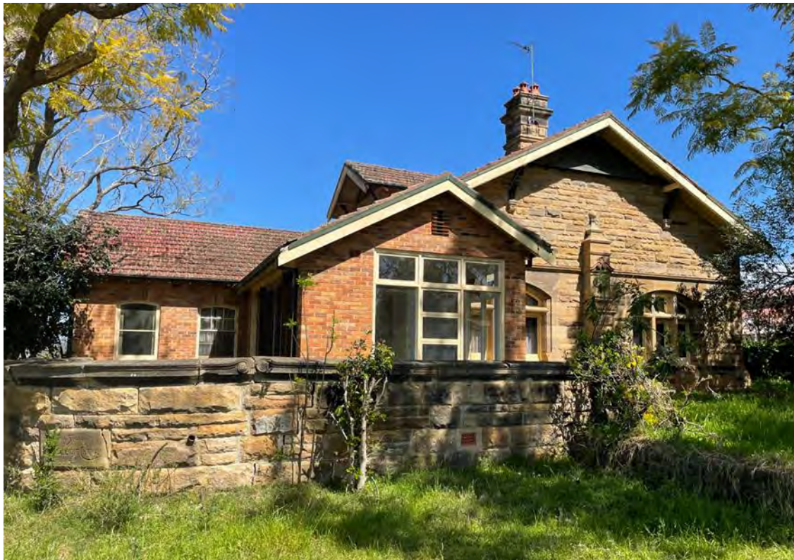
Plate 3-9: North eastern elevation of Building 1. Note commemorative stone in retaining wall at lower left (AECOM, 2022)
