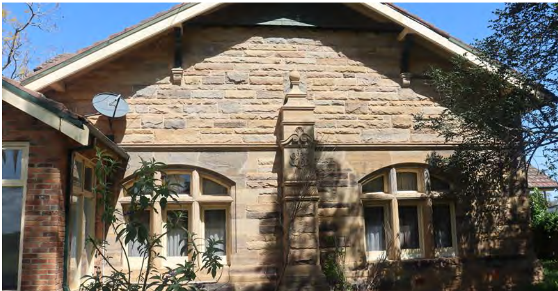
Plate 3-8: Finial in north-eastern elevation with the carving of entwined numbers "1896" (AECOM, 2022)
