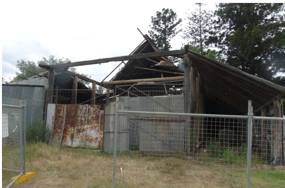
Figure 6. 7: Northern elevation of Tebbutts Barn in 2019
