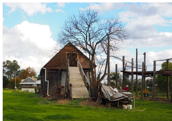
Figure 6. 4: Early 19 th century slab barn at No. 353 Pitt Town Bottoms Road, Pitt Town Bottoms with ramp access to loft.
