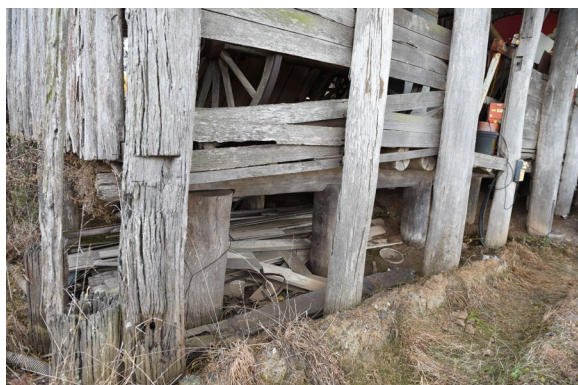
Figure 3. 35: Detail of floor structure to barn at 176B Hibberts Lane, Freemans Reach.
