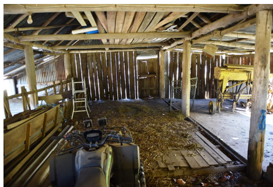
Figure 3. 38: Feed storage section of barn at No. 239 Upper MacDonald Road, St Albans.
