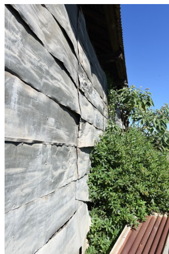
Figure 3. 30: Flat iron plates covering over original wall cladding to barn at No. 56 Freemans Reach Road, Freemans Reach.
