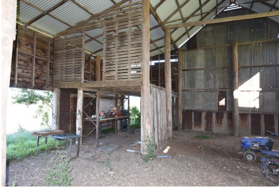
Figure 3. 17: Loft structure in skillion addition in barn at No. 353 Freemans Reach Road, Freemans Reach.
