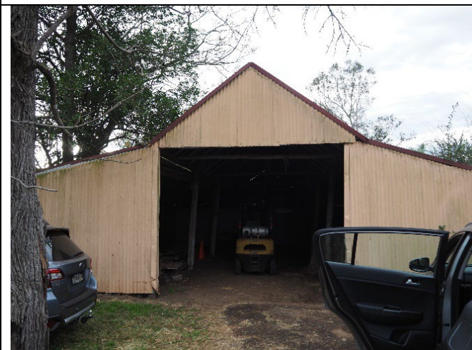
Caption: Barn2 at 141 Blacktown Road, Freemans Reach (exterior) Photographer: K. Denny Copyright Owner: Lucas Stapleton Johnson & Partners Date: June 2023
