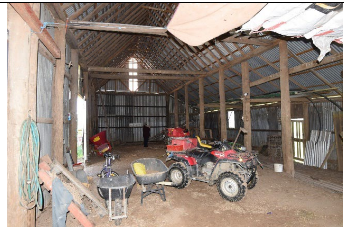
Caption: Barn B at 331 Freemans Reach Road, Freemans Reach (interior)
