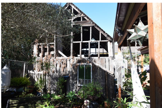
Figure 3. 10: Town barn at rear of No. 4 Catherine Street, Windsor.
