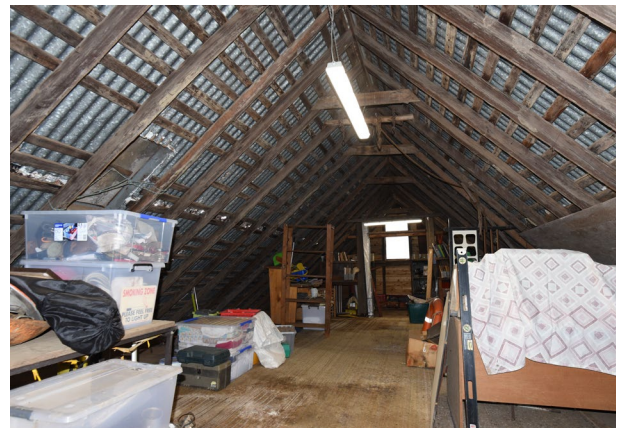
Figure 3. 27: Shingle battens with corrugated iron roof cladding to barn at No. 353 Pitt Town Bottoms Road, Pitt Town Bottoms
