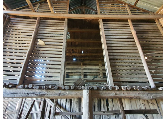
Figure 3. 18: Loft structure in barn at No. 87 Wilberforce Road, Wilberforce.
