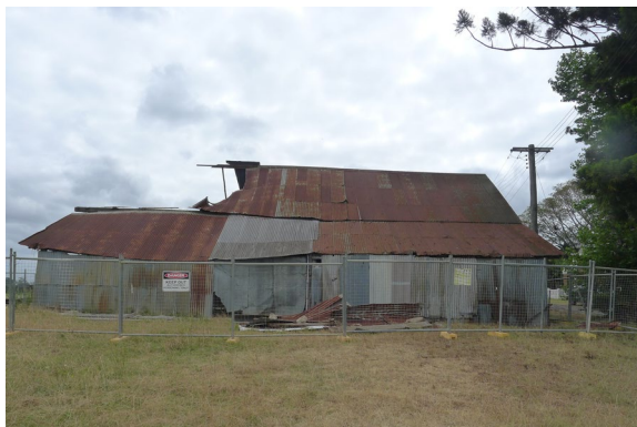
Figure 6. 8: Western elevation of Tebbutts Barn in 2019
