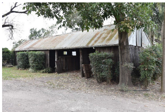
Figure 3. 22: Slab stables at No. 254 Yarramundi Lane, Agnes Banks
