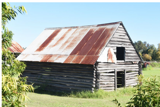
Figure 3. 21: The horizontal log outbuilding at No. 11 Amelia Grove, Pitt Town, which is possibly a corn drying shed.
