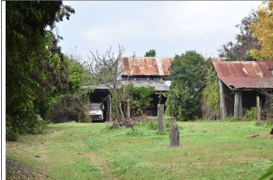
Caption: Barn at No. 2 Yarramundi Lane / 2 Old Kurrajong Road, Agnes Banks Photographer: S. Johnson Copyright Owner: Lucas Stapleton Johnson & Partners Date: June 2023
