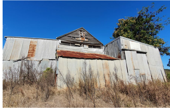
Figure 3. 32: Weatherboard infill to gable end of main barn at No. 87 Wilberforce Road including loft door.
