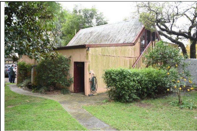
Caption: Barn 1 at 141 Blacktown Road, Freemans Reach (exterior) Photographer: K. Denny Copyright Owner: Lucas Stapleton Johnson & Partners Date: June 2023
