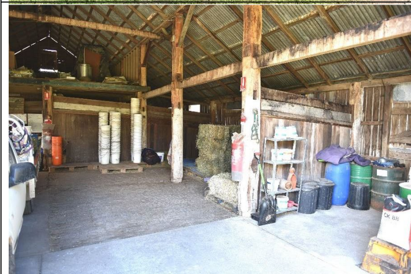
Caption: Barn 1 at 331 Hobartville, 36-40 Inalls Lane, Richmond (interior) Photographer: S. Johnson Copyright Owner: Lucas Stapleton Johnson & Partners Pty Ltd Date: June 2023
