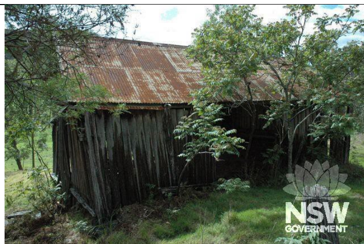
Caption: Slab barn at No. 1665 Upper Colo Road, Upper Colo. Photographer: C. Edds Copyright Owner: Graham Edds & Associates Date: 2010
