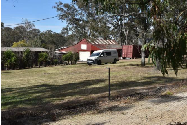
Caption: Barn at No. 331 Grono Farm Road, Wilberforce Photographer: S. Johnson Copyright Owner: Lucas Stapleton Johnson & Partners Date: July 2023
