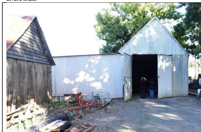
Caption: Barn A at 253 Wilberforce Road, Wilberforce (exterior) Photographer: S. Johnson Copyright Owner: Lucas Stapleton Johnson & Partners Pty Ltd Date: May 2023
