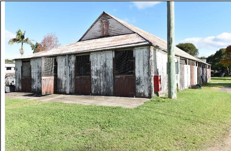
Caption: Barn 1 at 331 Hobartville, 36-40 Inalls Lane, Richmond (exterior) Photographer: S. Johnson Copyright Owner: Lucas Stapleton Johnson & Partners Pty Ltd Date: June 2023
