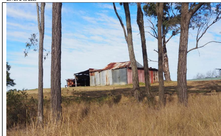
Caption: Barn at 8 Burdekin Road, Wilberforce (exterior) Photographer: K. Denny Copyright Owner: Lucas Stapleton Johnson & Partners Pty Ltd Date: July 2023
