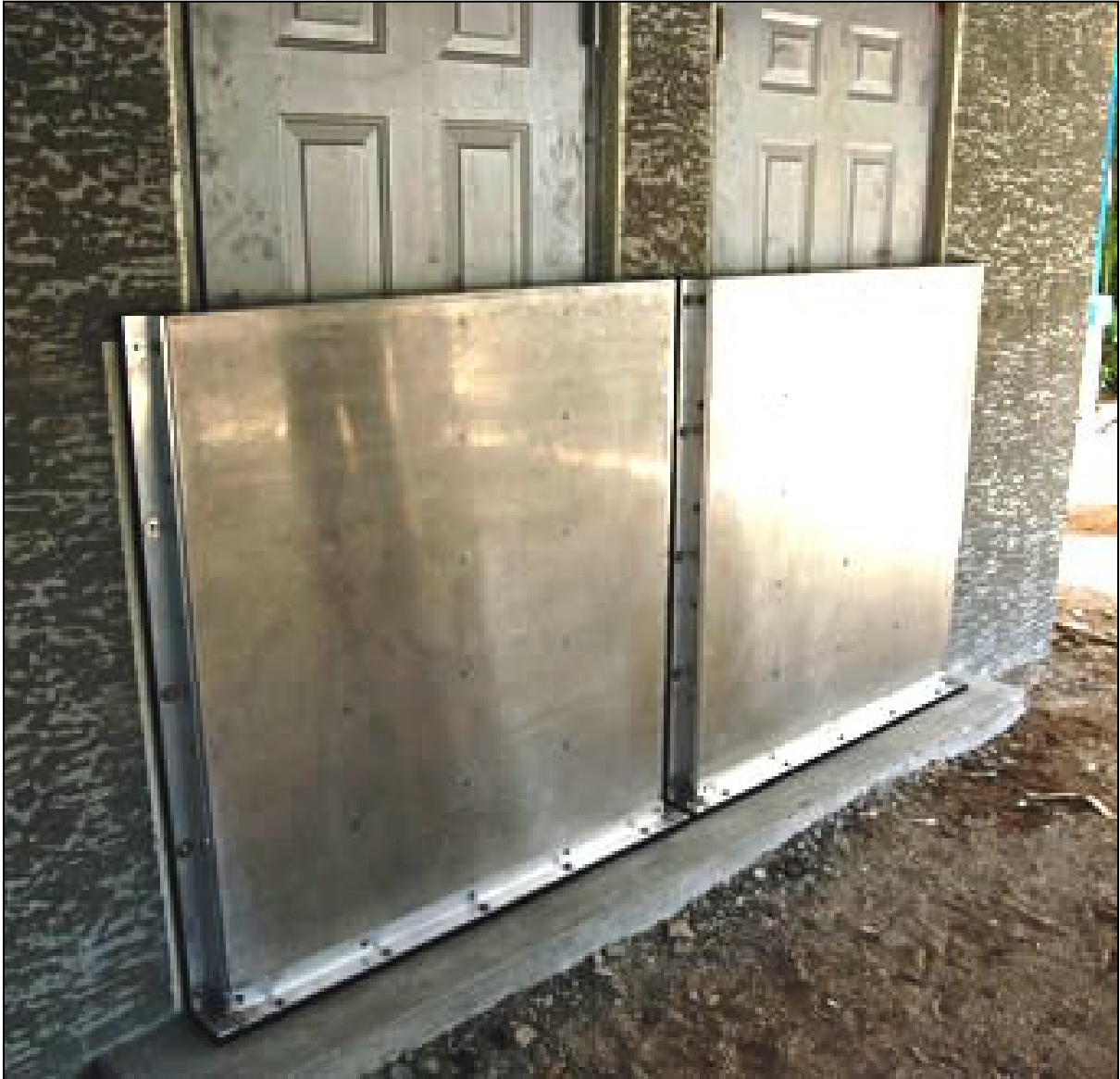
Photo 2: Dry proofing on doors of residential property
