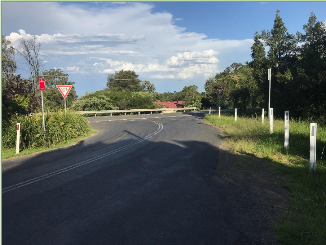
View looking east along Warks Hill Road at the intersection with Bells Line of Road
