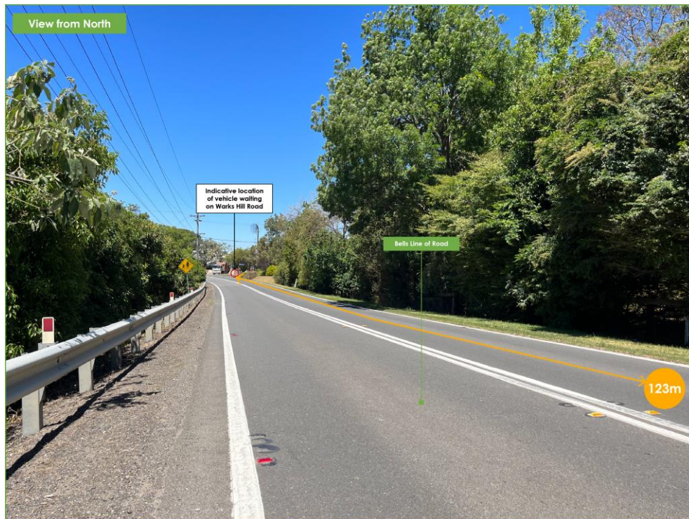
Figure 2: Warks Hill Road Sight Distance to Southbound Traffic (Approx. 123m)
