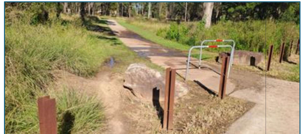
At another crossing, where riders have created their own bypass track.
