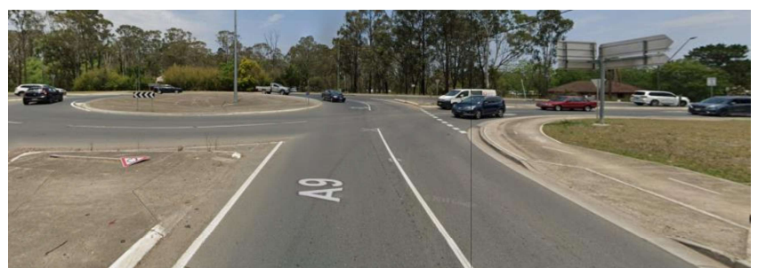
Google Street View image of looking back at the Richmond Rd roundabout from near the George St shared path crossing. Two lanes of turning traffic from the left and one lane from the right can make it difficult to judge when safe to cross.
