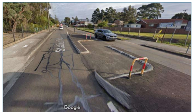
Google Street View image of the 'offset refuge' on Station St, Toongabbie.
