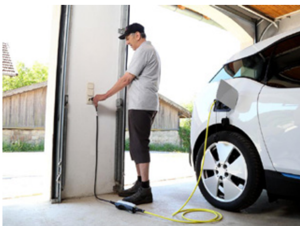
Figure 15: Making homes EV ready
