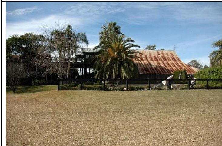
Caption: Barn A at No. 265 Pitt Town Bottoms Road, Pitt Town Bottoms Photographer: C. Edds Copyright Owner: Grahams Edds & Associates Date: 2009
