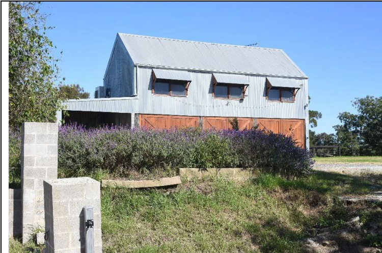
Caption: Barn at 123 Freemans Reach Road, Freemans Reach (exterior) Photographer: S. Johnson Copyright Owner: LSJ Heritage Date: May 2023
