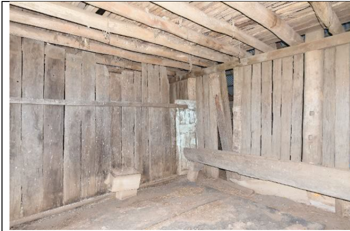
Caption: Barn A at 331 Freemans Reach Road, Freemans Reach (interior) Photographer: LSJ Copyright Owner: Lucas Stapleton Johnson & Partners Pty Ltd Date: May 2023
