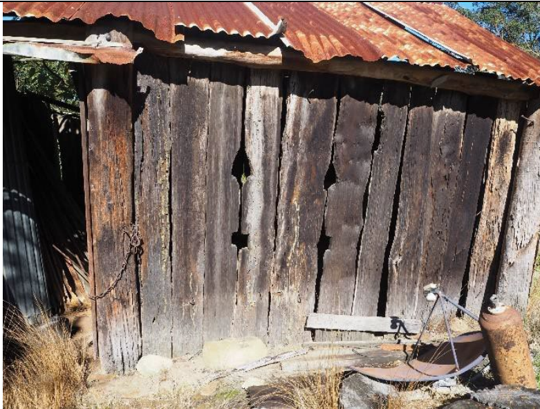
Caption: Slots for rails in slab wall of stables at 480 Laws Farm Road, Lower Portland Photographer: S. Johnson Copyright Owner: Lucas Stapleton Johnson & Partners Date: June 2023
