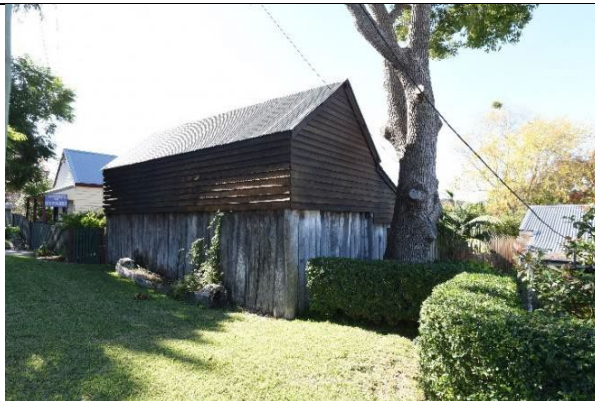
Caption: The town barn at No. 4-8 Chatham Street, Pitt Town Photographer: S. Johnson Copyright Owner: Lucas Stapleton Johnson & Partners Date: May 2023
