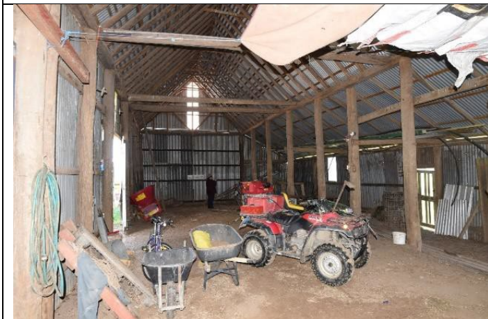
Caption: Barn B at 331 Freemans Reach Road, Freemans Reach (interior) Photographer: LSJ Copyright Owner: Lucas Stapleton Johnson & Partners Pty Ltd Date: May 2023
