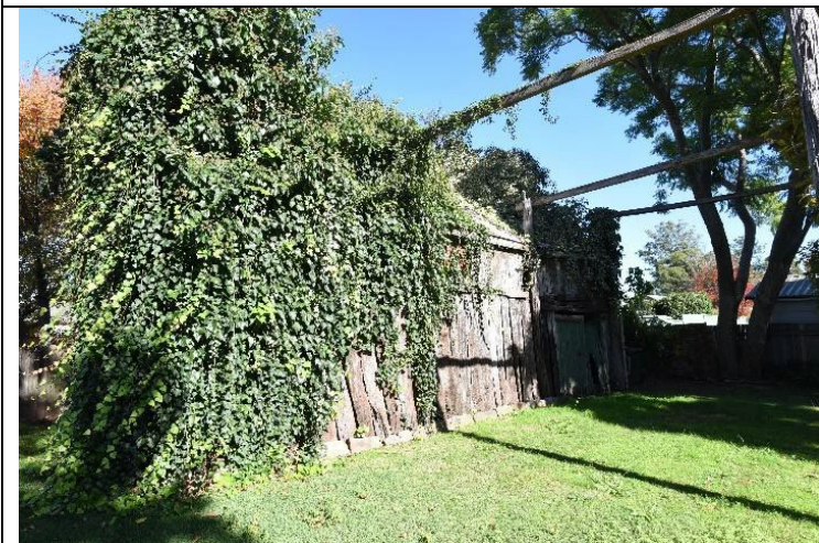
Caption: Barn 2 at No. 20-22 Buckingham Street, Pitt Town Photographer: S. Johnson Copyright Owner: Lucas Stapleton Johnson & Partners Date: May 2023
