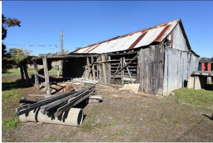
Caption: Former blacksmith workshop and house at No. 292 Pitt Town Road, Pitt Town (exterior) Photographer: S. Johnson Copyright Owner: Lucas Stapleton Johnson & Partners Date: May 2023
