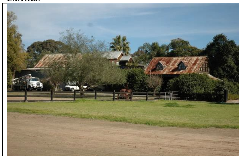
Caption: Barns at No. 265 Pitt Town Bottoms Road, Pitt Town Bottoms Photographer: C. Edds Copyright Owner: Grahams Edds & Associates Date: 2009
