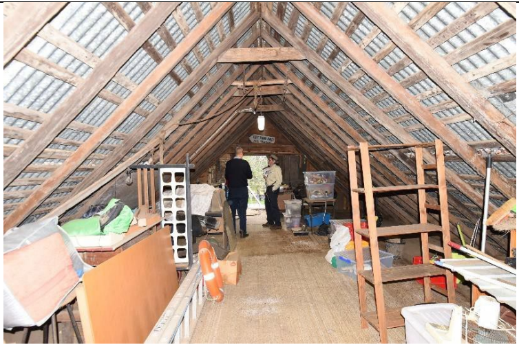
Caption: Barn at No.353 Pitt Town Bottoms Road, Pitt Town Bottoms (interior of loft) Photographer: S. Johnson Copyright Owner: Lucas Stapleton Johnson & Partners Pty Ltd Date: May 2023
