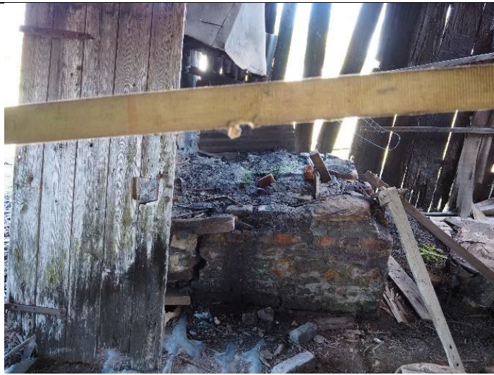
Caption: Brick hearth inside former blacksmith workshop at No. 292 Pitt Town Road, Pitt Town Photographer: S. Johnson Copyright Owner: Lucas Stapleton Johnson & Partners Date: May 2023
