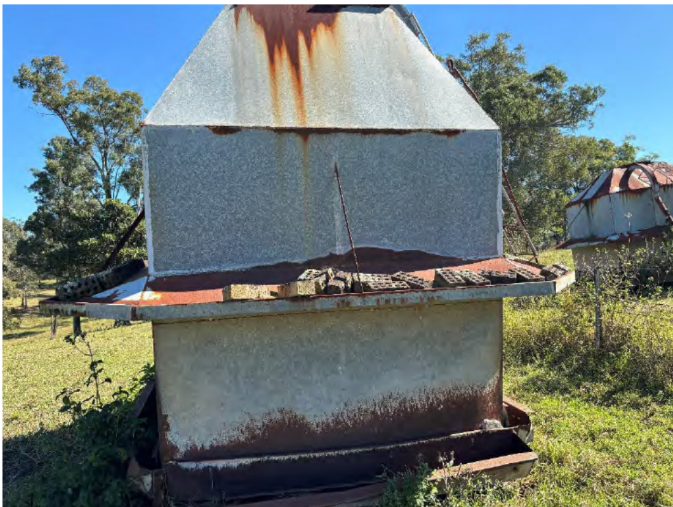
PHOTO 2 Redundant cattle grazing infrastructure
