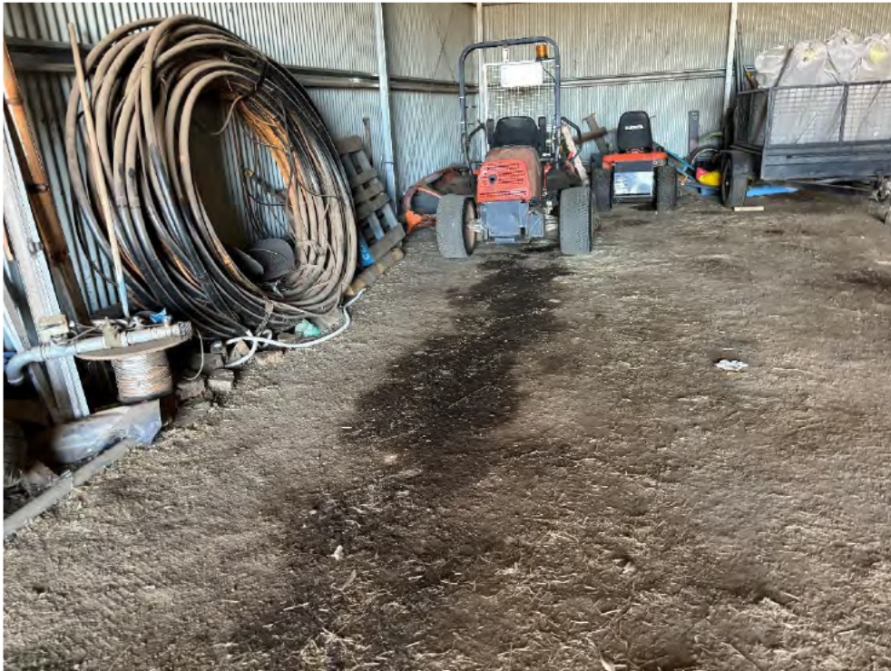
PHOTO 9 Observed staining on the inside of the tin shed.
