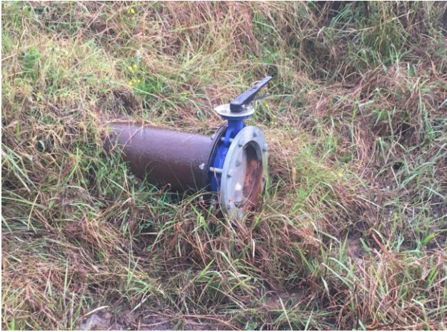
Figure 11 Detail of replaced outlet valve at Dam 3.
