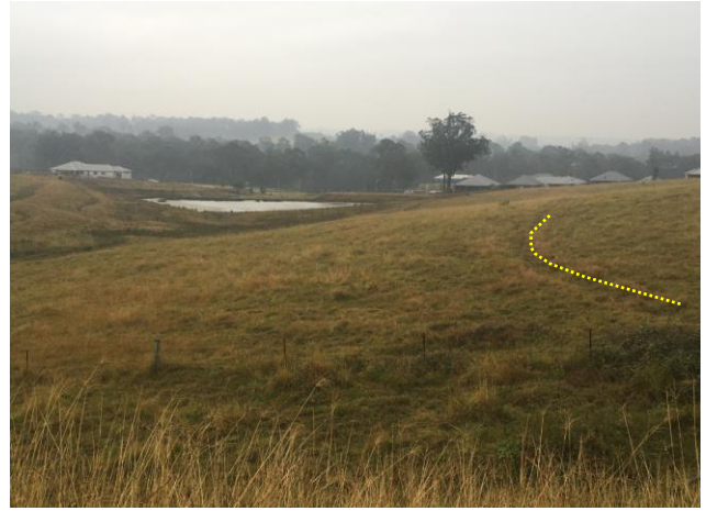
Figure 12 Valley view towards dam 11 with remnant drain indicated at right.
