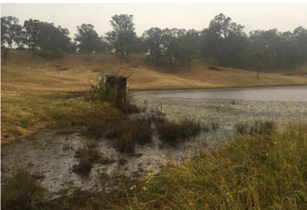
Figure 9 Remnant feeder swale from dam 3.
