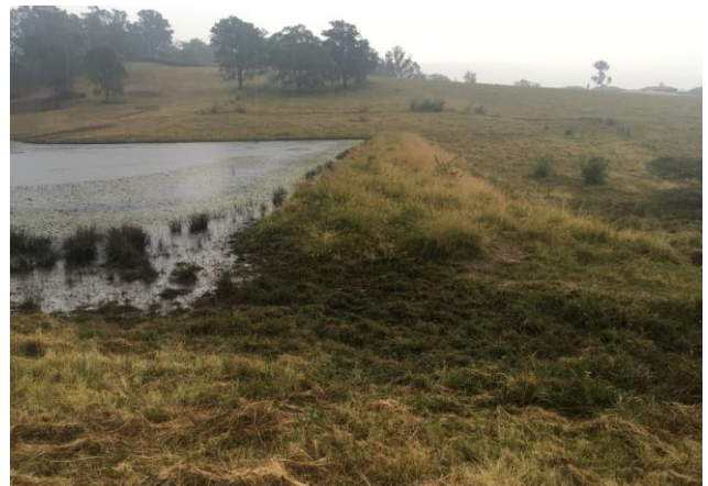
Figure 8 View of the dam wall (dam 3).
