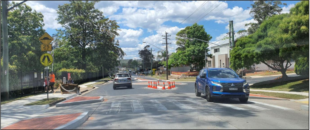
Figure 12 Roundabout at the Grose Vale Road / Sunnyside Crescent intersection (Source: Site visit, November 2022)
