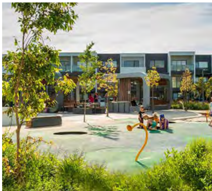
Jack Road Town Houses, VIC
