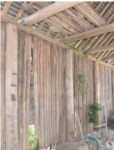
Figure 3. 28: Detail of palisade wall cladding and shingle battens to barn at No 56 Freemans Reach Road, Freemans Reach.
