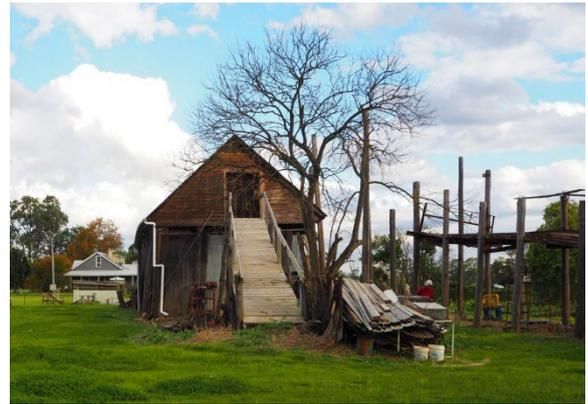
Figure 6. 4: Early 19<sup>th</sup> century slab barn at No. 353 Pitt Town Bottoms Road, Pitt Town Bottoms with ramp access to loft.
