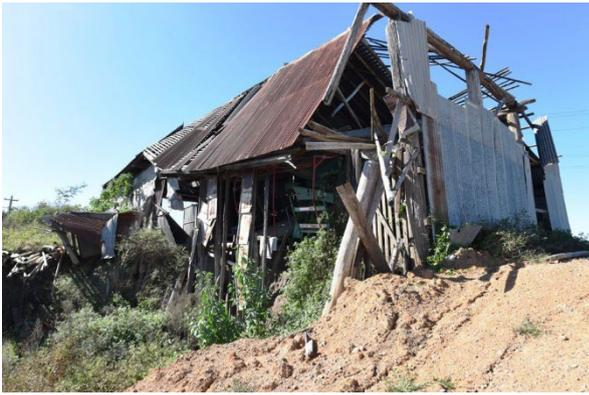
Figure 6. 3: Early 19<sup>th</sup> century slab barn at No. 56 Freemans Reach Road, Freemans Reach showing the impacts of 2022 floods on the structure as a result of the washing away of river bank.
