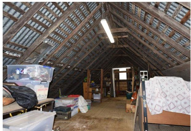
Figure 3. 27: Shingle battens with corrugated iron roof cladding to barn at No. 353 Pitt Town Bottoms Road, Pitt Town Bottoms
