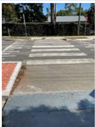
Figure 24: Zebra crossing outside Richmond North Public School
