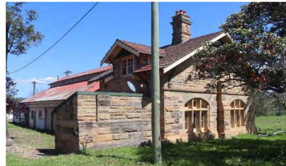
Plate 3-20: Building 2, looking south (AECOM, 2022)
