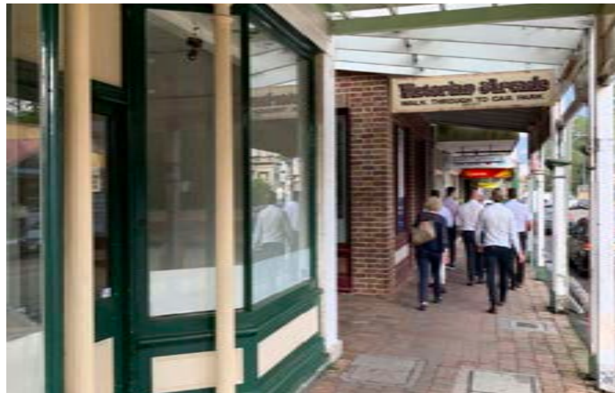
Awning providing shade to pedestrians along Windsor Street
