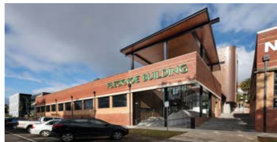
Adaptive re-use building
