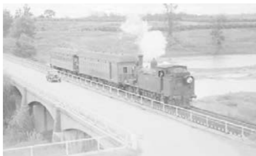
Car and Steam train crossing Richmond Bridge, Hawkesbury River, c. 1945, photograph by E.W. Searle. (Source: National Library of Australia, PIC P838/926a LOC Cold Store SEA Box)
