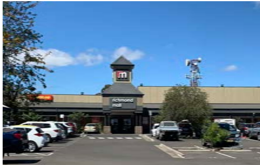
Richmond Mall main entrance off the parking lot has detracted activity from Windsor Street
