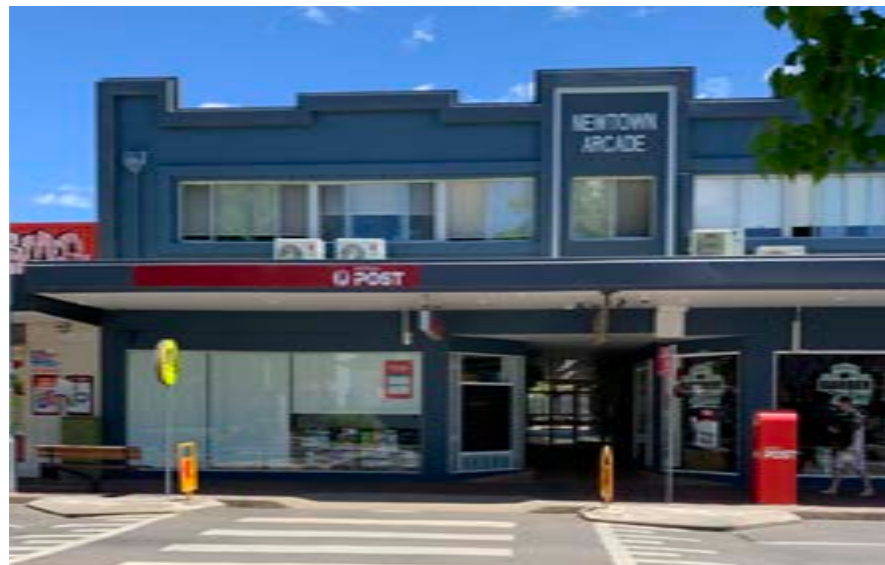
George Street streetscape with safe pedestrian crossing
