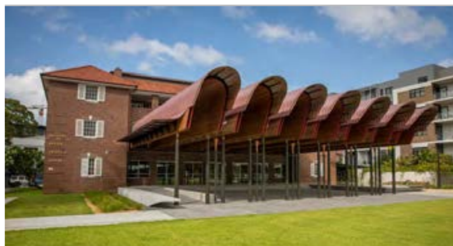
Adaptive re-use and fit out to heritage building
