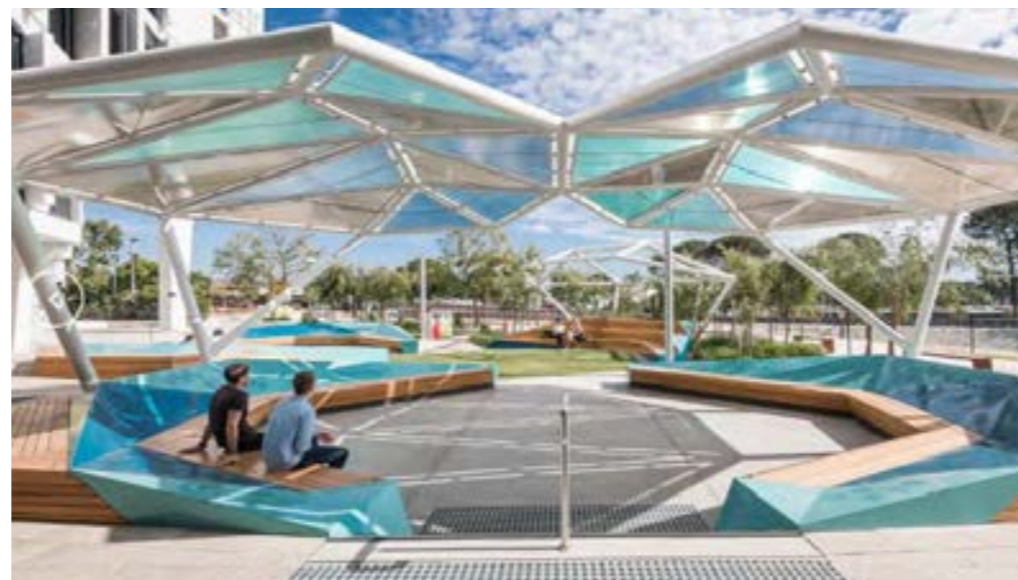
Seating pod and structure
