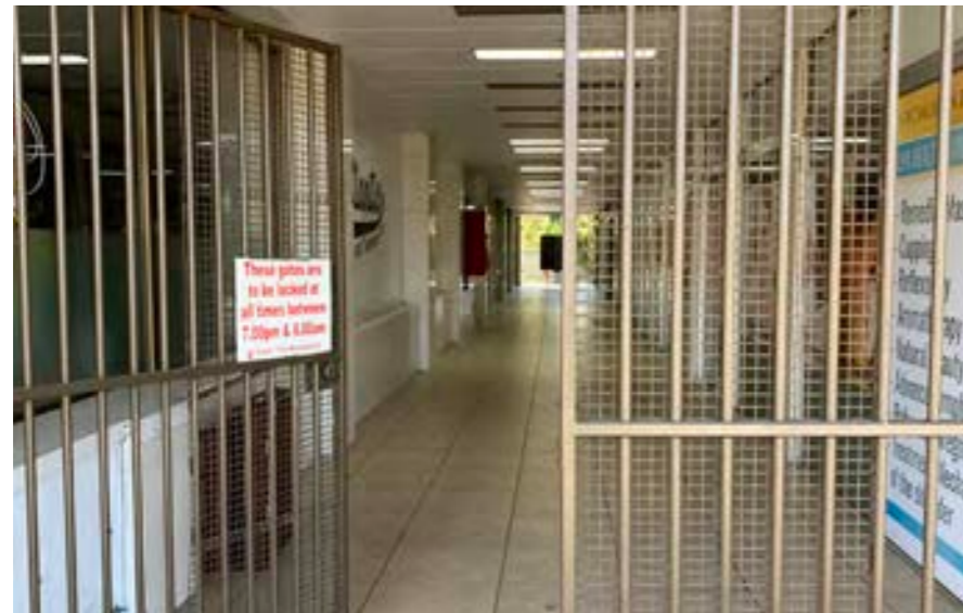
Under-utilised arcade connecting George Street and Mullinger Lane
