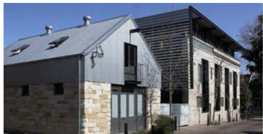
Adaptive re-use building
