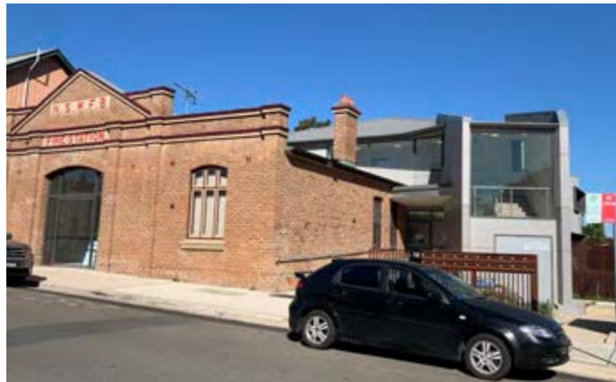
Recently completed project in Windsor adjacent to heritage site.
