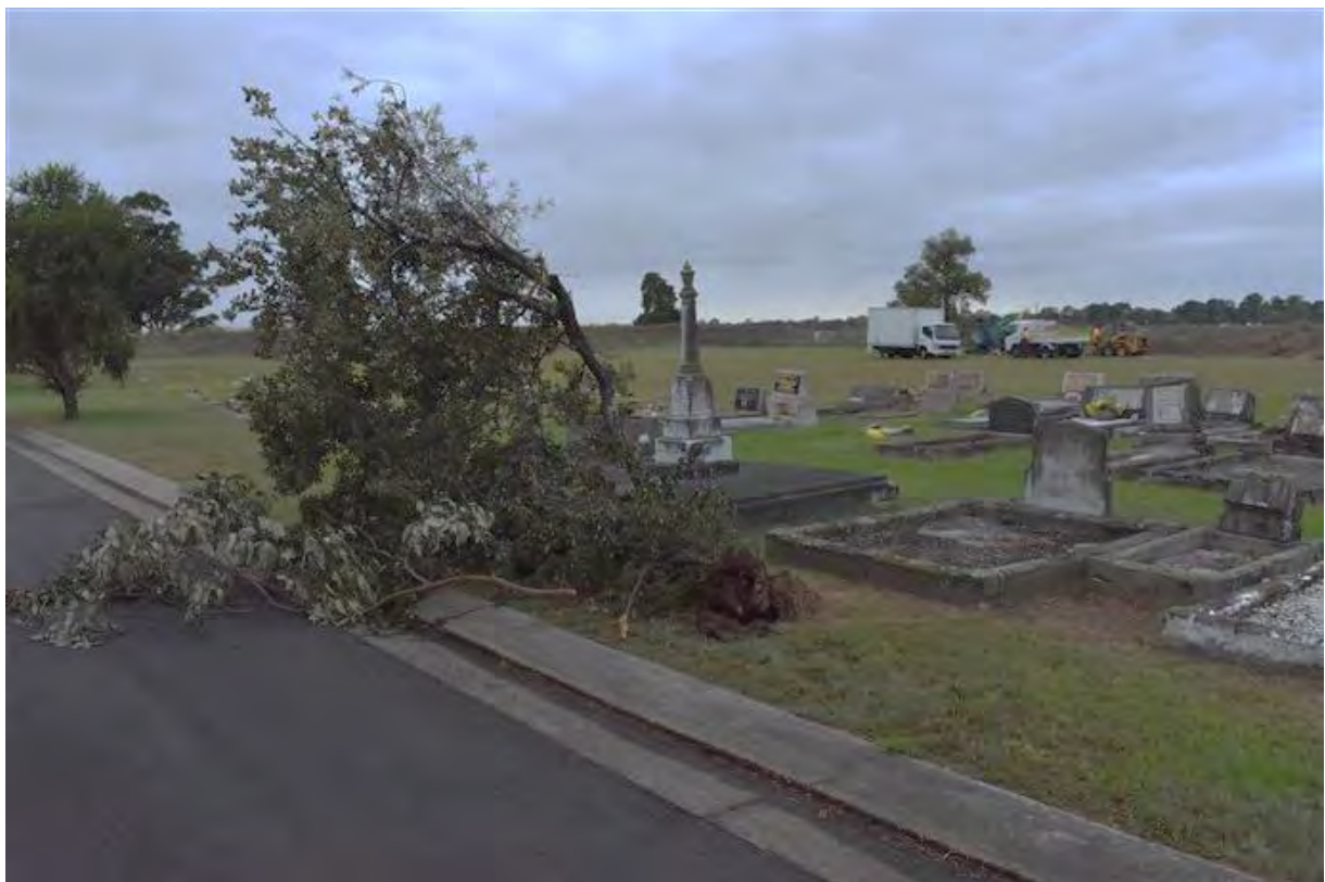
Figure 8 View looking south showing low kerb with a fallen tree, possibly from vehicle impact, in the central, older burial area of the cemetery. (Source: GML Heritage, 2019)
