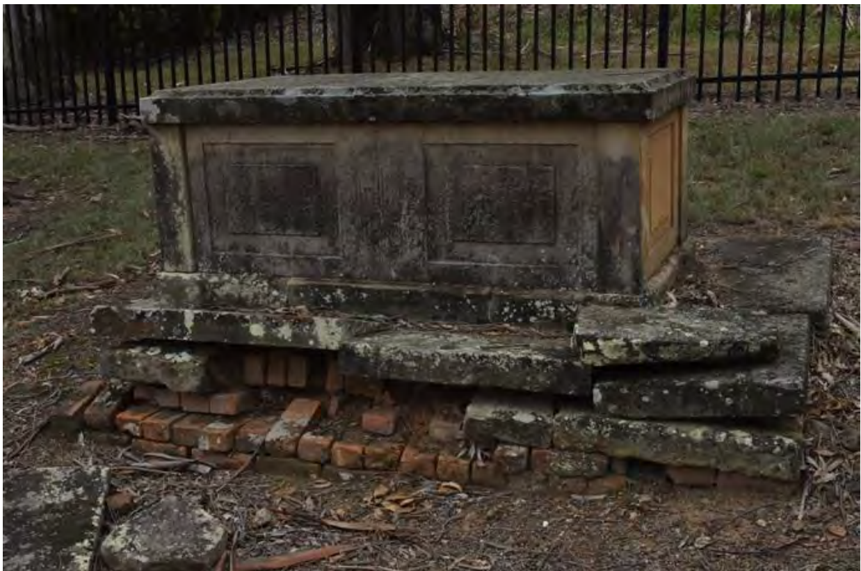
Figure 7 Example of a table-style slab burial in existing poor condition. (Source: GML Heritage, 2019)
