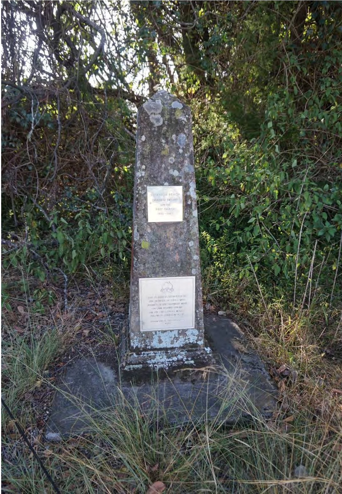
Figure 13 Sandstone obelisk marking the site of the former St Thomas' Anglican Church. (Source: GML Heritage, 2019)
