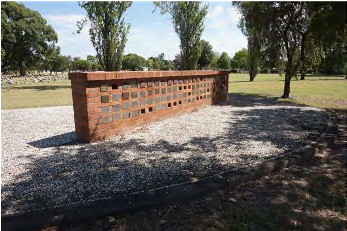
Figure 10 Brick columbarium adjacent to entrance. (Source: GML Heritage, 2019)
