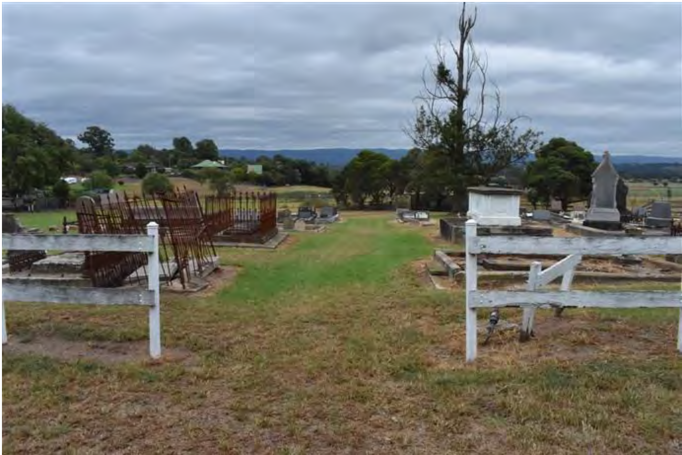
Figure 4 View looking west through the cemetery entrance. Note the wrought iron grave surround on left, likely impacted by a vehicle. (Source: GML Heritage, 2019)
